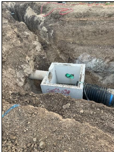
Site Storm Drain
