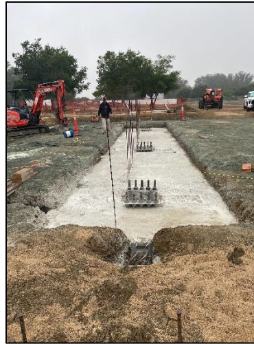
Grade Beam Concrete
