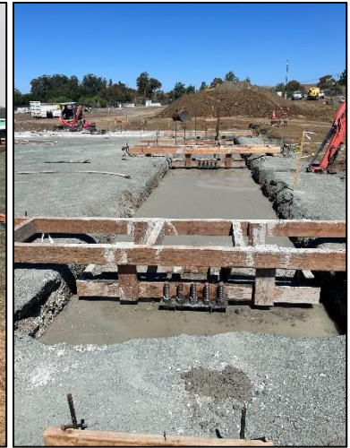
Grade Beam Concrete
