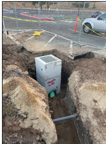
Site Storm Drain
