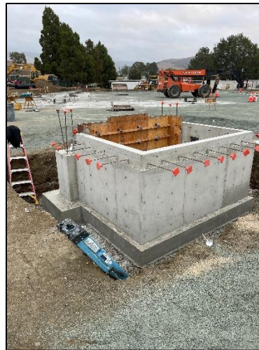
Elevator Pit Wall Concrete
