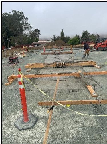
Grade Beam Concrete
