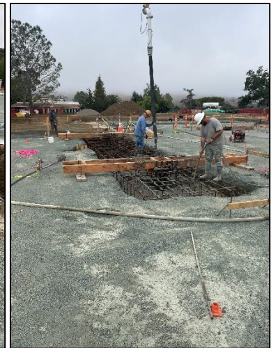
Grade Beam Concrete
