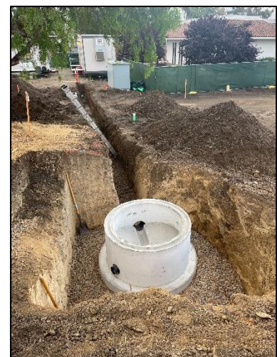
Site Sewer Trench to P.O.C.
