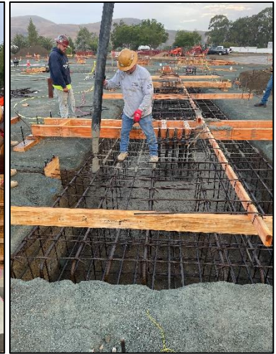
Grade Beam Concrete
