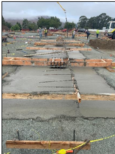
Grade Beam Concrete
