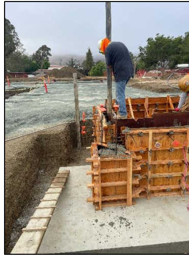
Elevator Pit Wall Concrete
