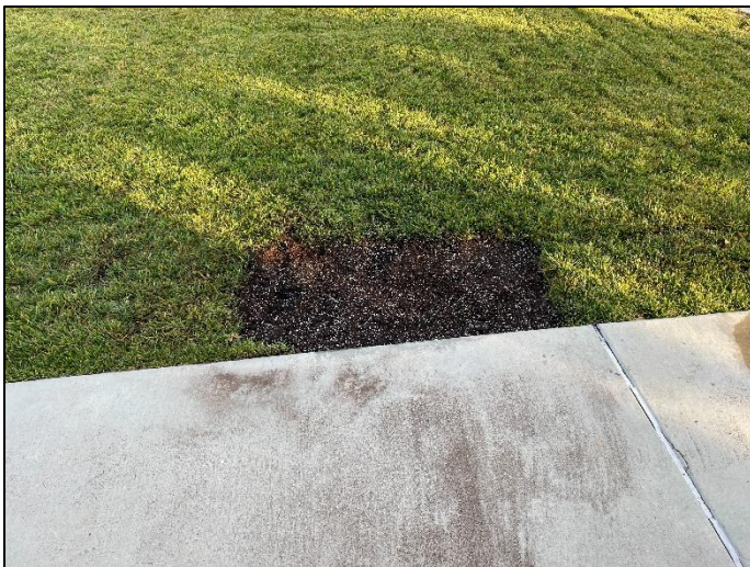
Footing Removed/Area Reseeded
