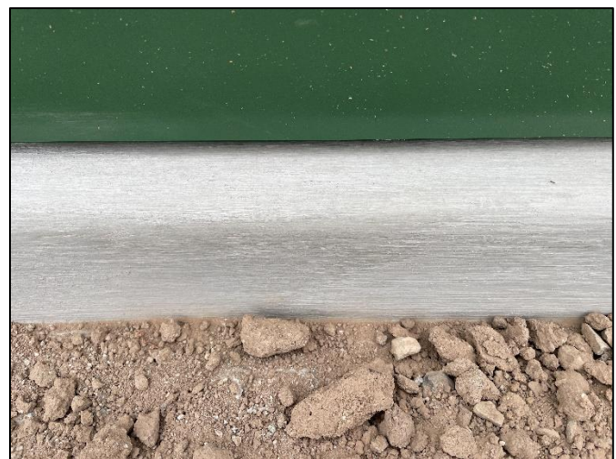
Retouched Footing Finish
