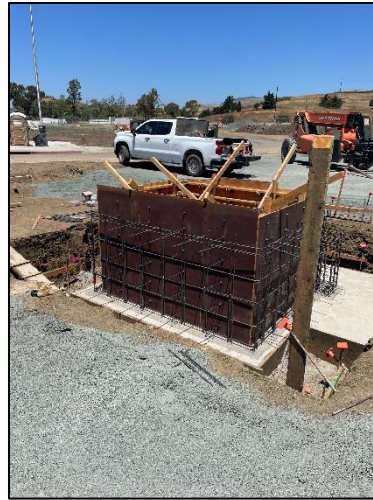
[ Elevator Pit Wall Rebar ] [ Elevator Pit Wall Formwork ]
