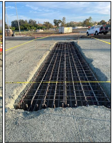
[ Building Grade Beam ]
