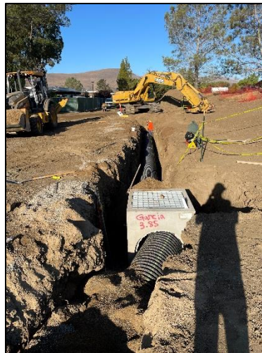
[ Site Storm Drain Piping ]
