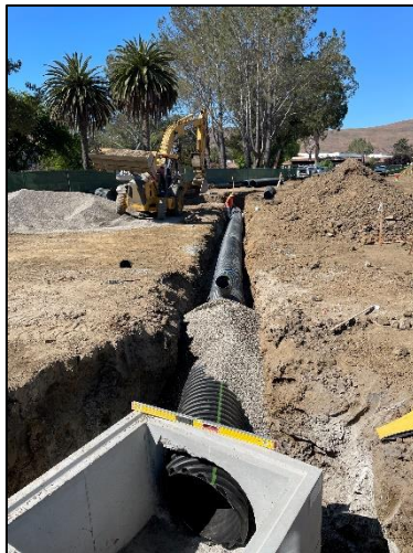
[ Site Storm Drain Piping ]
