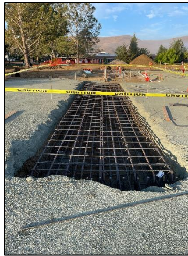
[ Building Grade Beams ]
