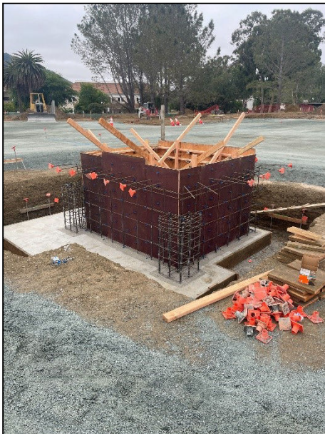
Elevator Pit Wall Forms
