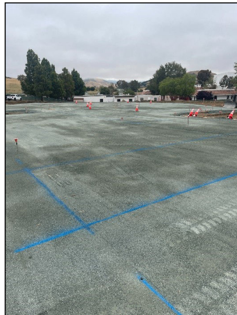
Grade Beam Markings
