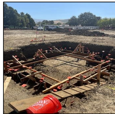
Formed Elevator Pit
