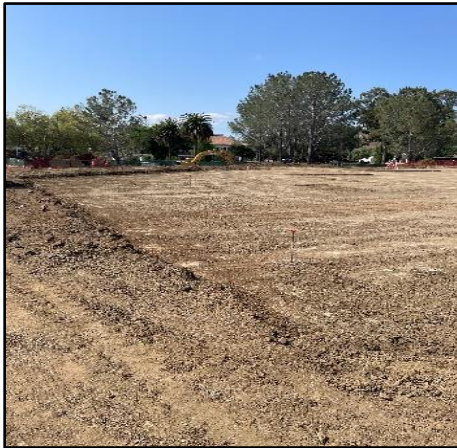
Fully Compacted Building Pad
