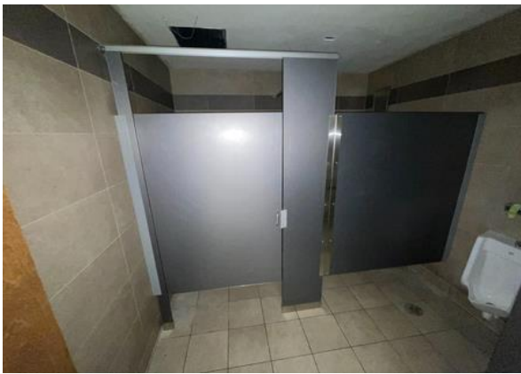
Building 6200 Men's Restroom
