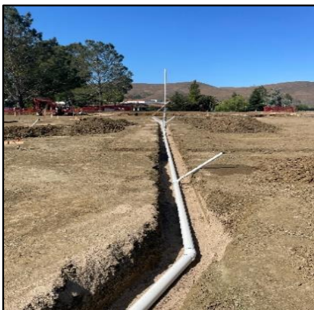
Underground Utility Installation
