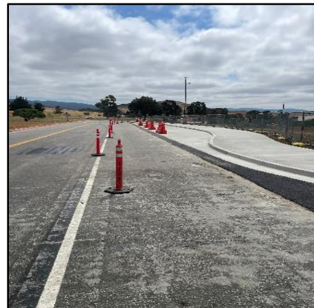
New Bus Stop Turnout
