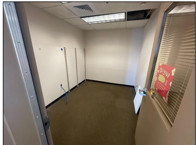
New cable pulled to data ports
