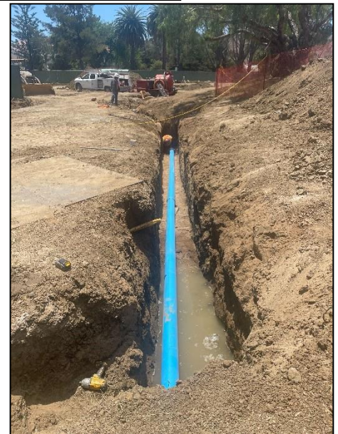
Water Line Installation
