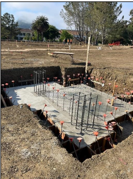
Elevator Pit Concrete
