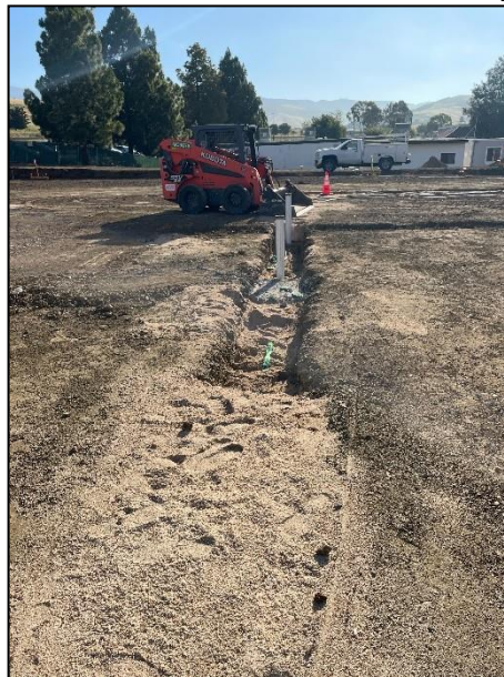
Trench Backfill
