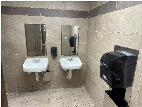
Sinks & RR Accessories Installed
