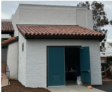
Tile Roof Complete
