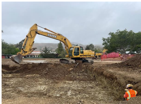
Building Pad Over Excavation
