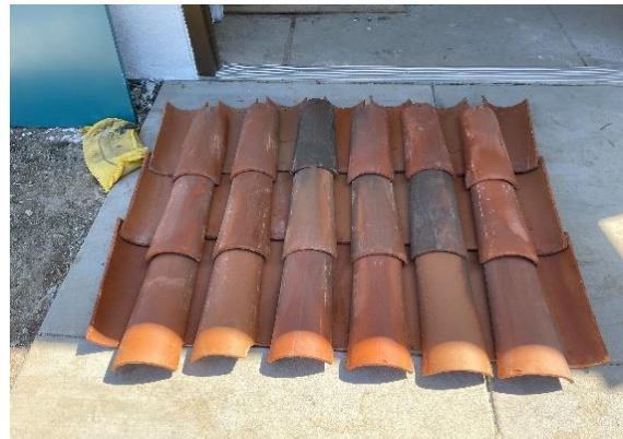
Tile roof mockup
