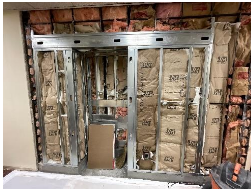
Framing/Insulation Bldg. 6200 DF alcove
