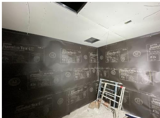
Moisture barrier Bldg. 6200 restrooms
