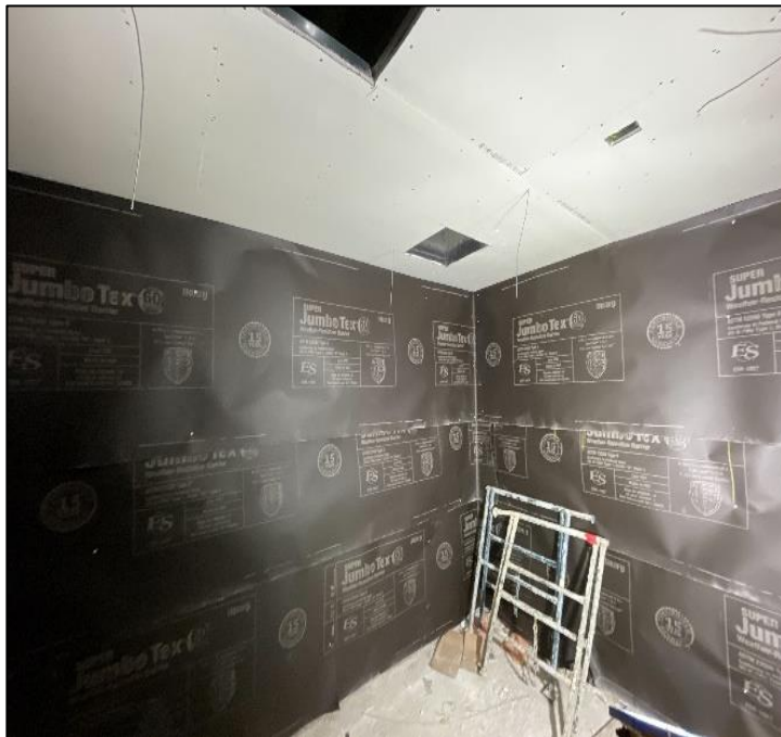
Vapor barrier in preparation for lath
