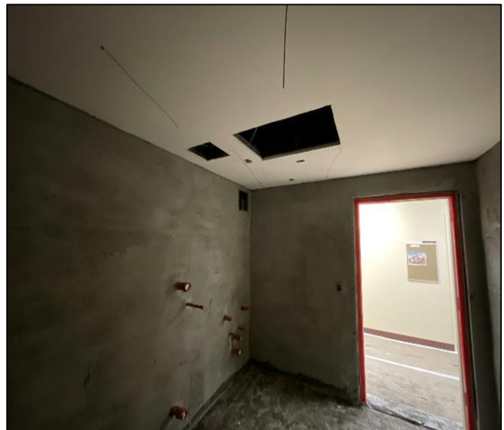
Plaster installed in preparation for tile
