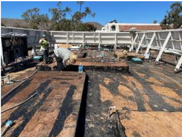
Demo of Existing Roofing/HVAC on Building 7100
