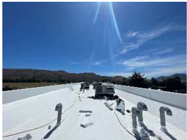
New Single Ply Roofing on Building 4000
