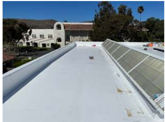
New Roofing Install for Building 7100 in Progress
