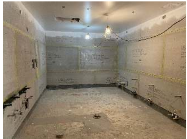
Building 7100 Restroom Progress
