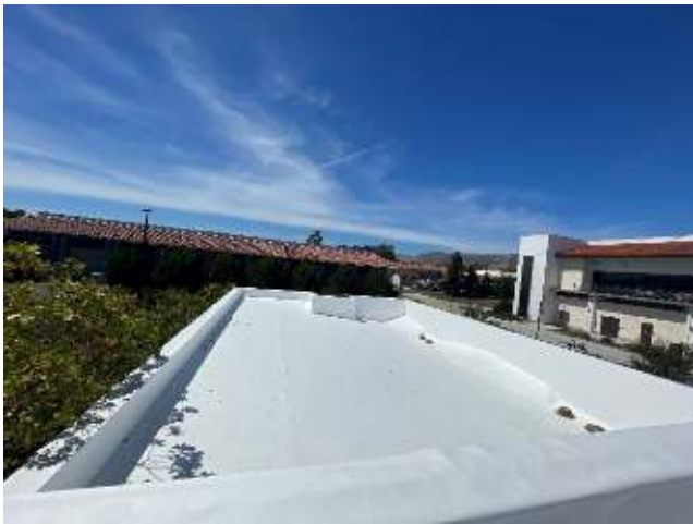
New Single Ply Roofing on Building 4000
