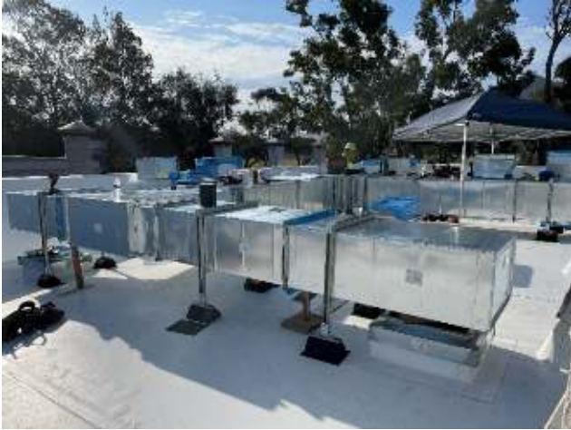
New Ductwork
