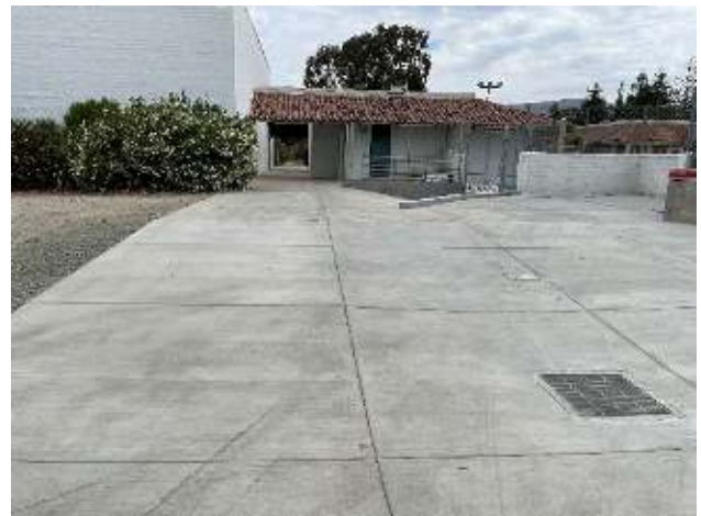
Additional Site Flatwork
