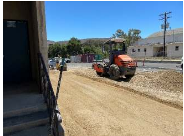
Base Compaction
