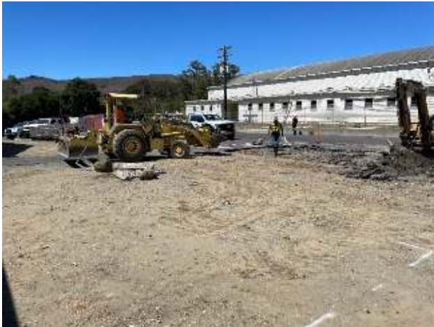
Demo of Existing Parking Lot
