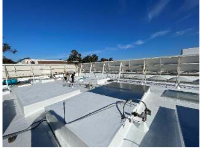
Sheet Metal Cap Installation
