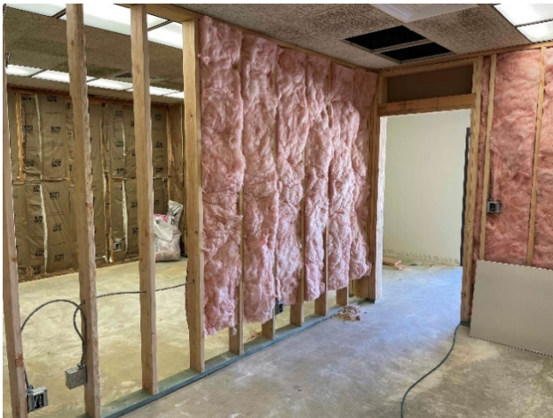
Wall Framing & Insulation
