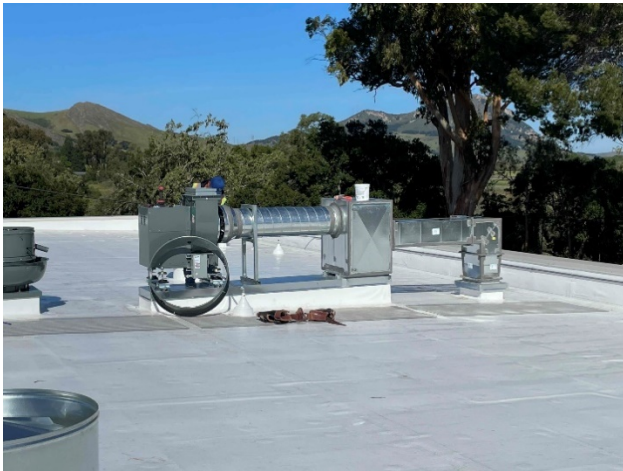
New Vehicle Exhaust Fans
