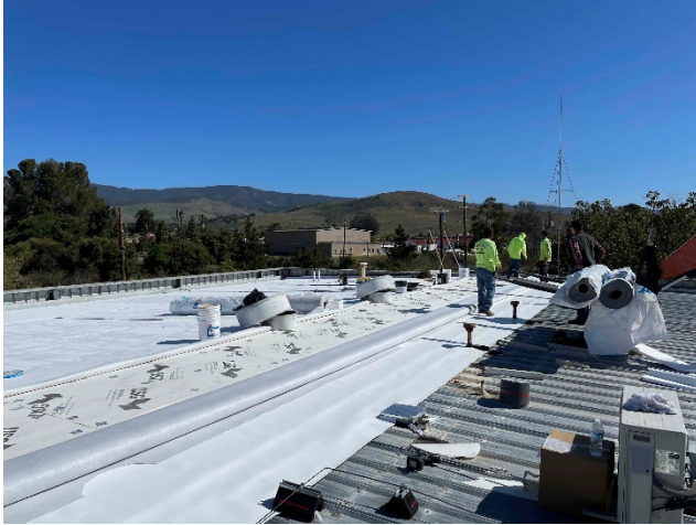
PVC Roofing Installation
