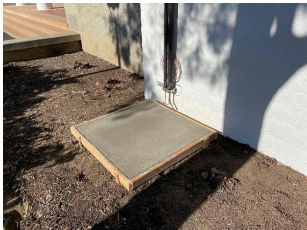
New Pad for Heat Pump
