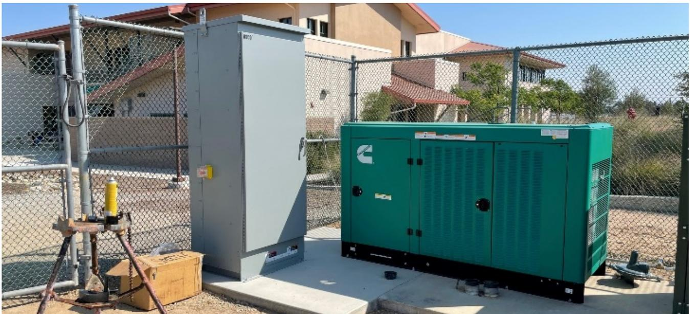
New Generator and MTS Installed on Concrete Pad at Chiller Yard
