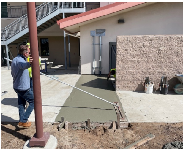
Concrete Placement at Walkway South of N3200
