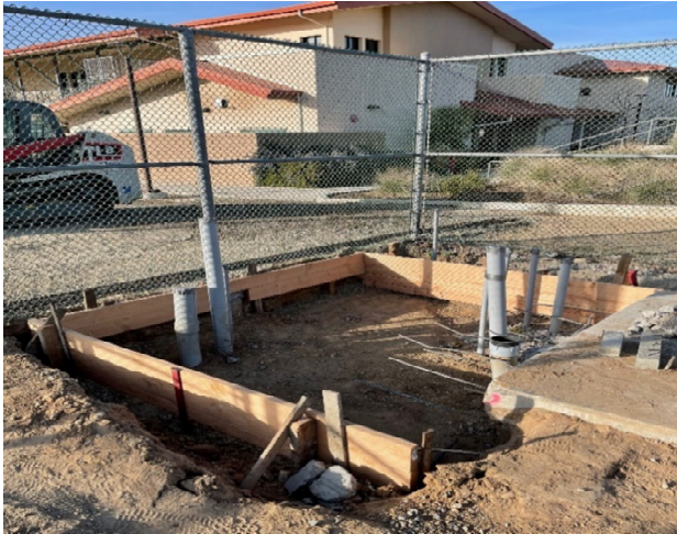
Conduit Stub-ups at the Concrete Generator Pad
