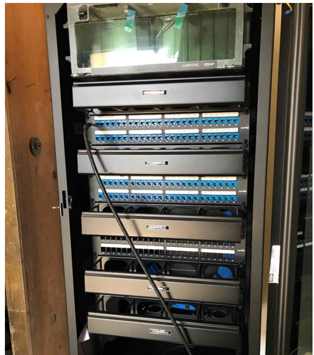
Installation of new Telecom Room Network Cabinet
