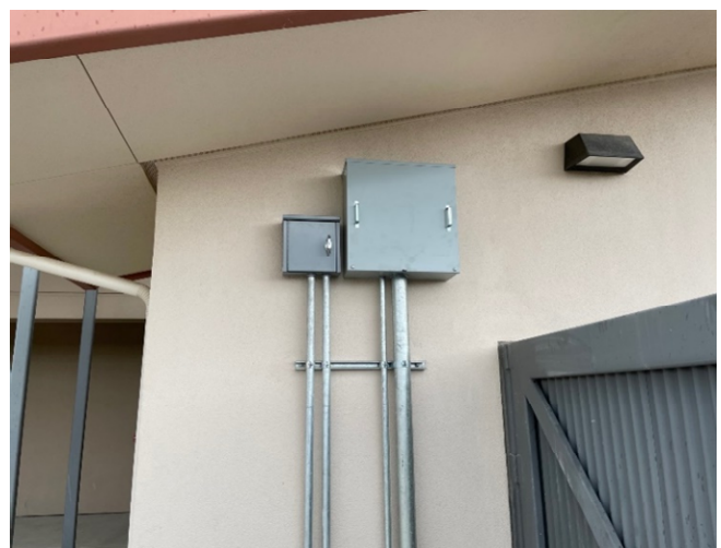
New Conduit Installed into the N3200 Data Center
