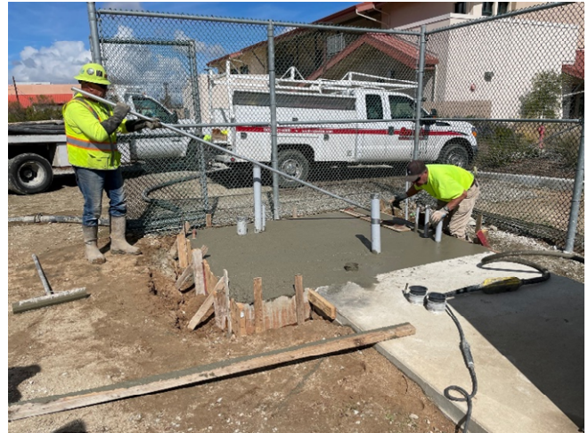
Concrete Placement for the New Generator Pad
