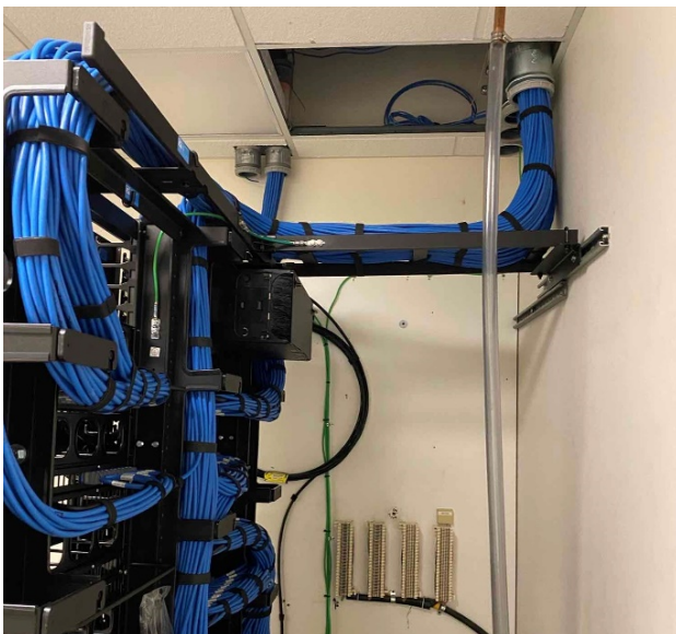
Installation of new Cat 6a cabling
