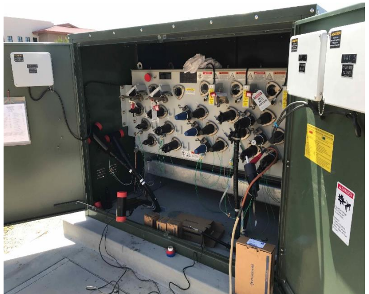
New Electrical Switchgear Installed
