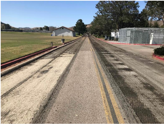
Asphalt Grinding at the Service Road and Parking Lot 5
