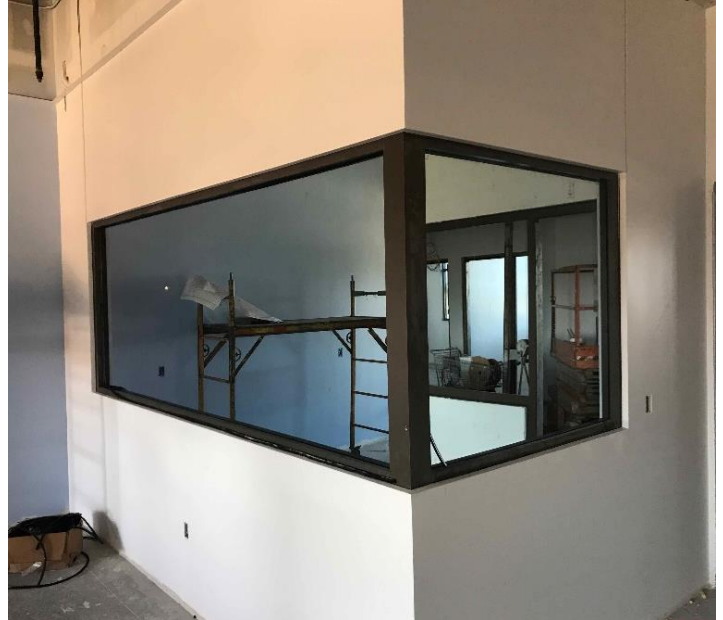
Observation Room One Way Glass Installed
