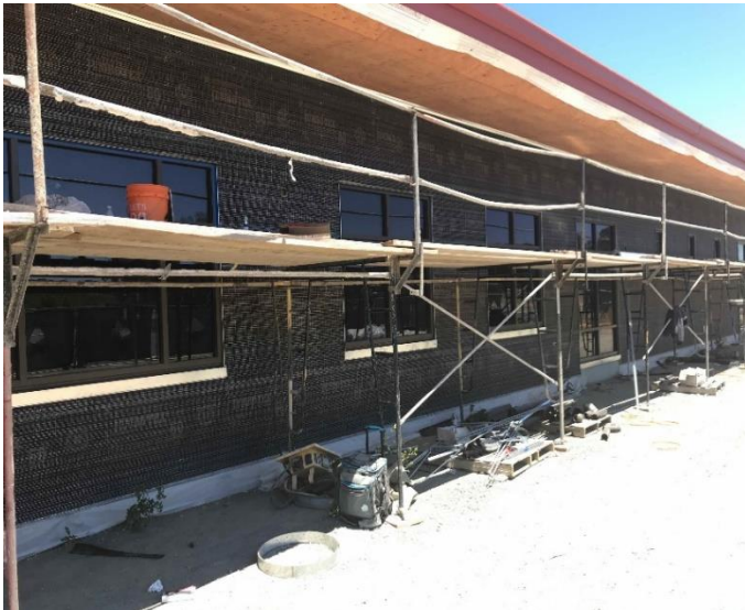
Exterior Lath Progress
