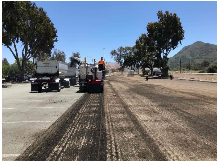
Asphalt Grinding at the Service Road and Parking Lot 5
