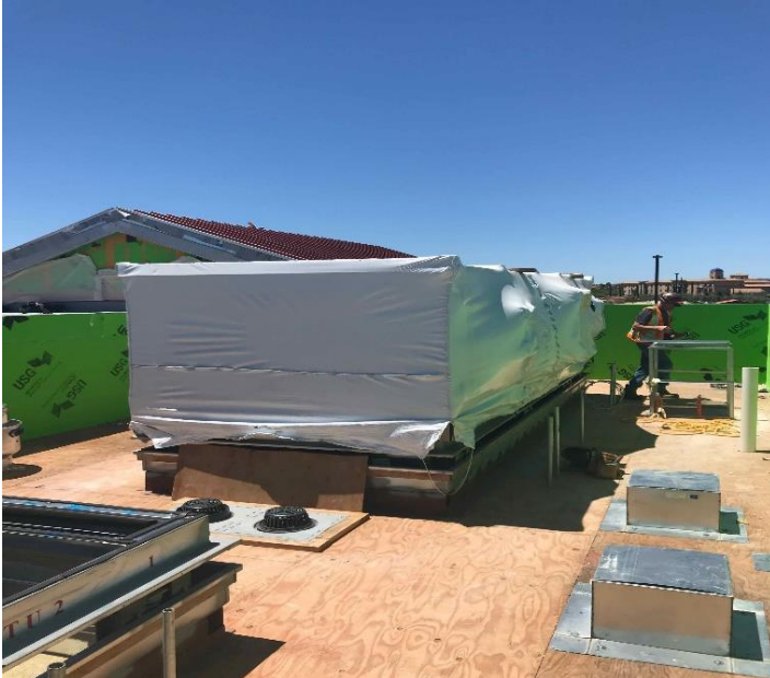
New HVAC Equipment Installed on Roof Curbs
