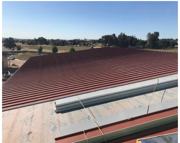
Installation of Standing Seam Metal Roof
