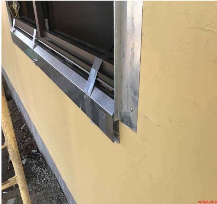
Window Installation Progress
