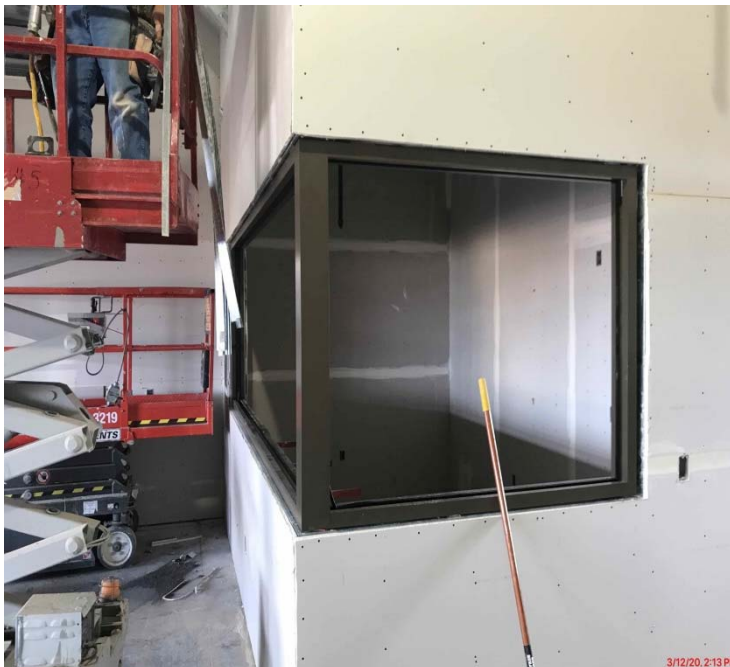
Interior Window Frames Installed
