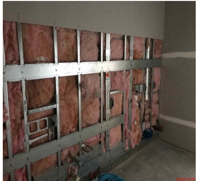
Insulation Installation Progress
