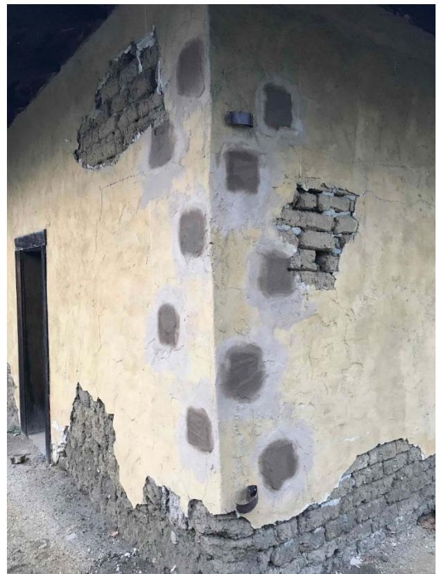
Patch back of Fiberglass Rods and Plates
