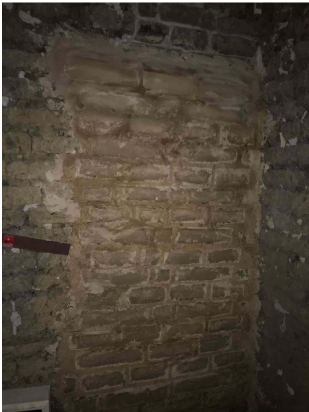
Door Infill Completed
