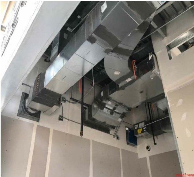
Ductwork Rough-in Complete
