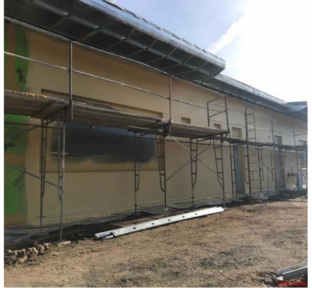
Installation of Weather Barrier
