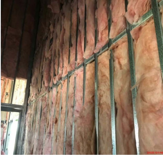
Insulation Installation
