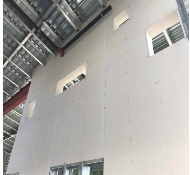
Exterior Sheathing Installation
