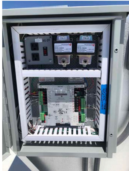
New HVAC Unit Controls
