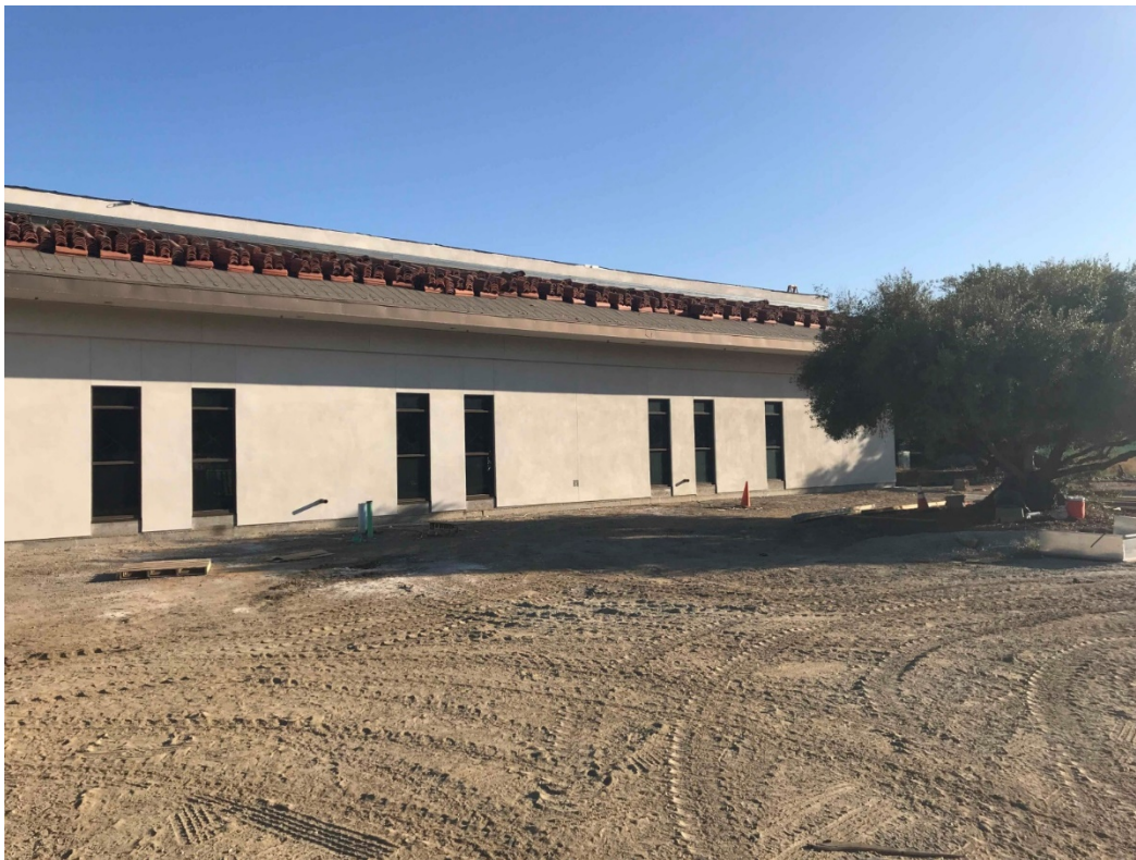
Data Center Exterior – Plaster Complete and Roof Tile Loaded
