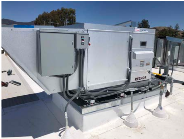
New HVAC Units and Final Connections
