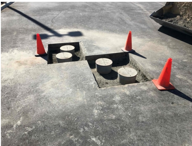
Valve Box Concrete Block-outs
