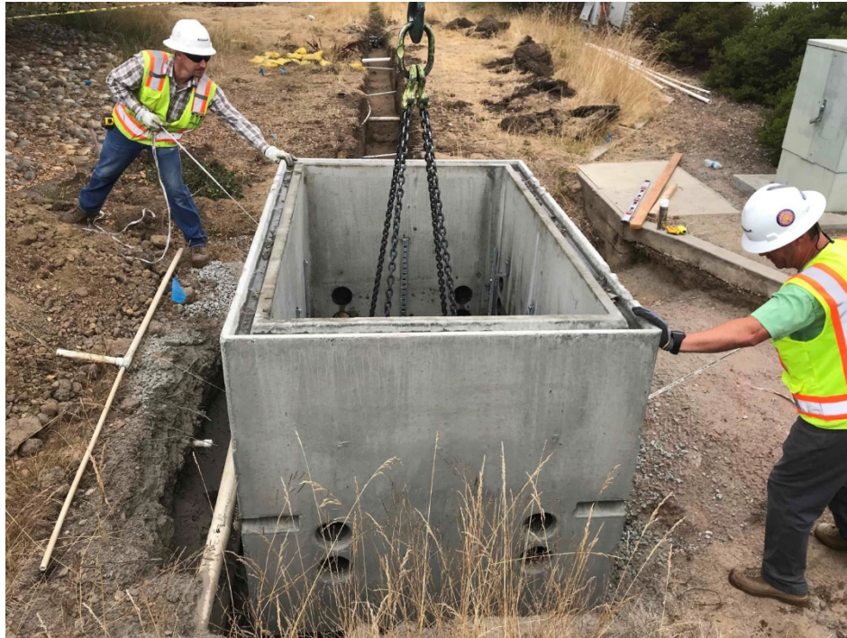
East Site Telecom Vault Installation
