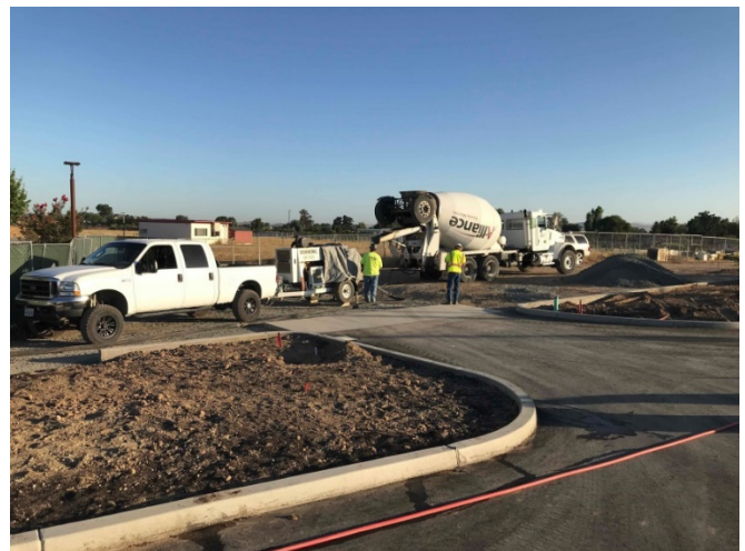
Concrete Curb & Gutter
