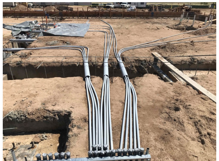
Underslab Utilities (Electrical)
