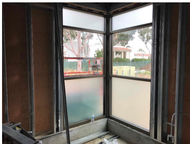
Window Frame and Glazing Installation
