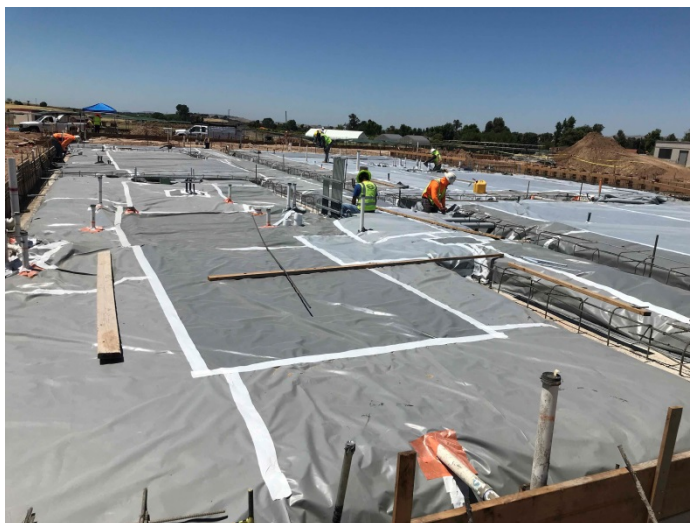
Vapor Barrier Installation
