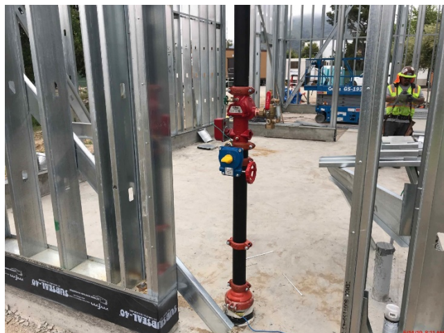
Fire Sprinkler Standpipe
