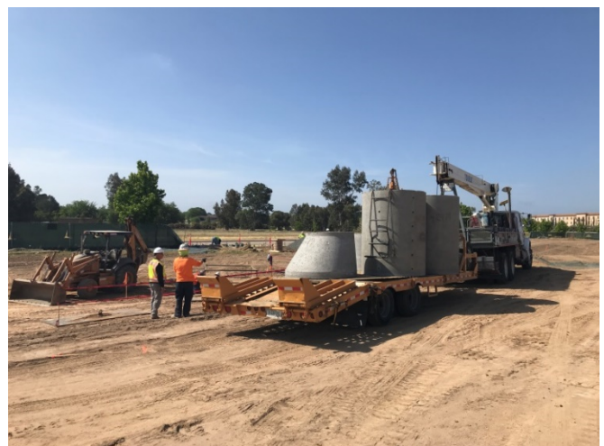
Storm Drain Manhole Delivery
