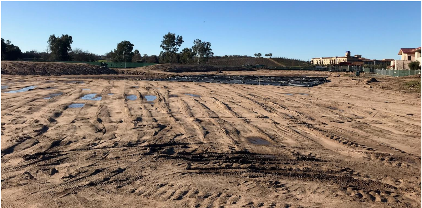
Overall Site Grading
