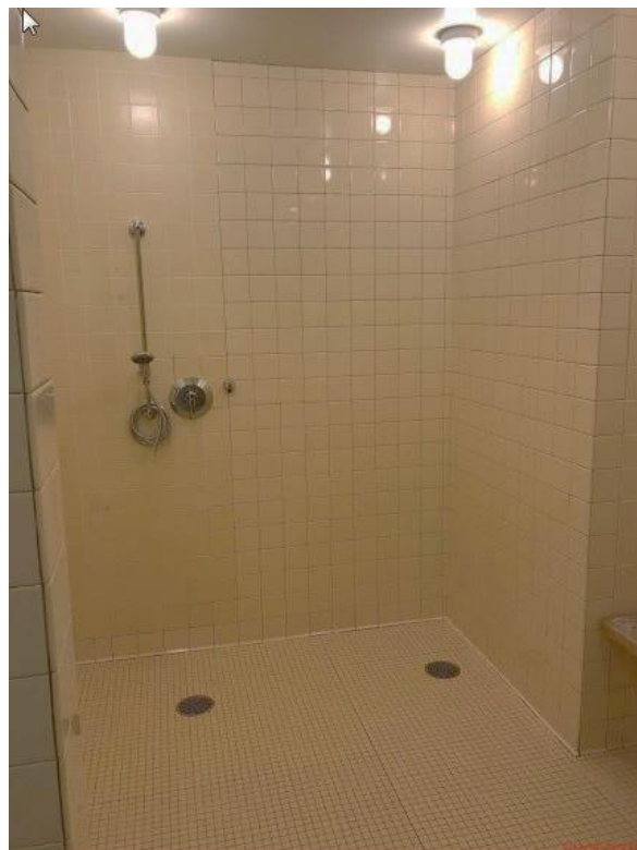
Shower in Men's Staff Locker room building 1100
