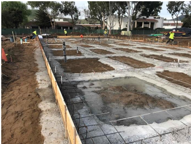
Placement of Concrete Grade Beams
