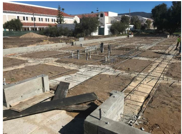
Completion of Concrete Structural Curbs
