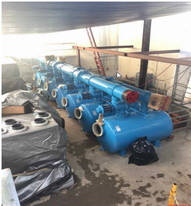
Pool Equipment Room Install Progress
