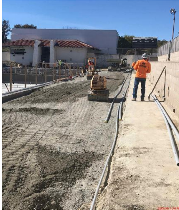
Concrete deck subgrade preparation around Competition Pool
