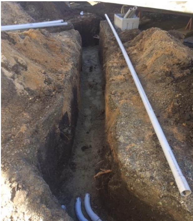
Underground Electrical install at 9100/9200
