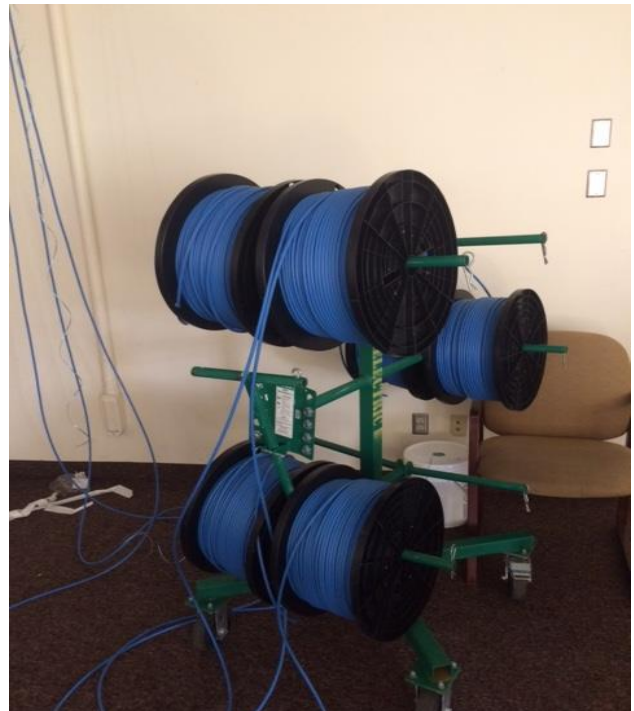
New Cabling install in 7400/7500
