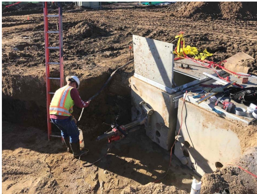
Main Electrical System Install
