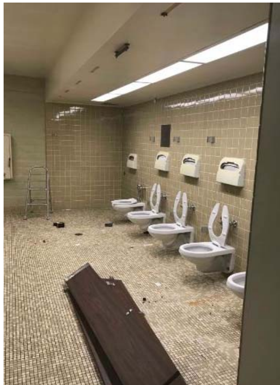
Building 1400 ADA Restroom Demo
