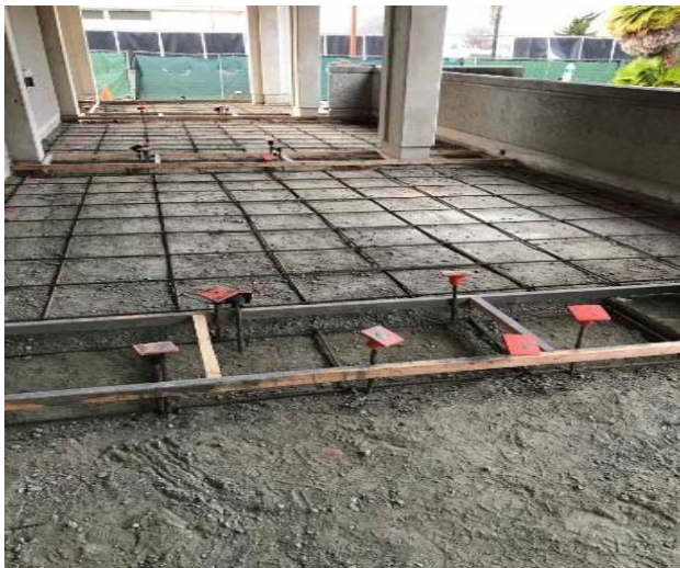
Building 1100 ADA Walkway
