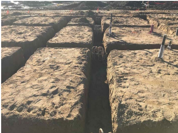
Trenching and Rebar for Grade Beams
