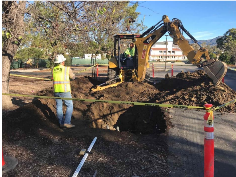
Main Sewer Line Connection at Lot 5
