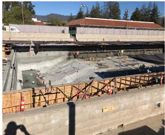
Competition Pool Concrete/Shotcrete Complete
