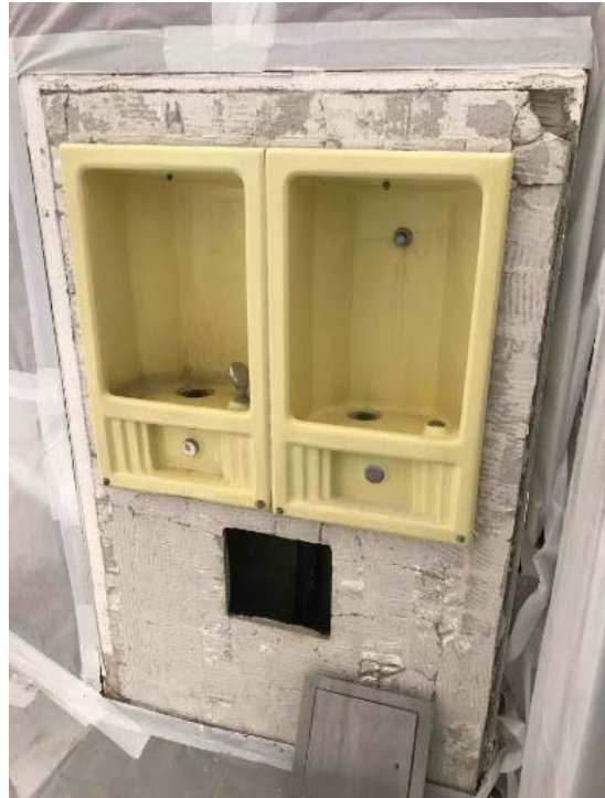
Building 1200 Removal of Drinking Fountains
