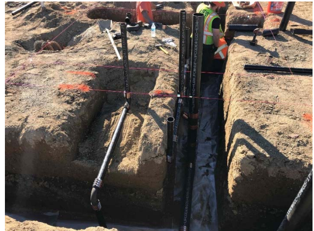
Underground Utility Install
