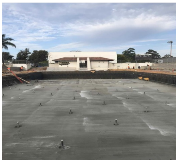
Competition Pool Concrete Floor
