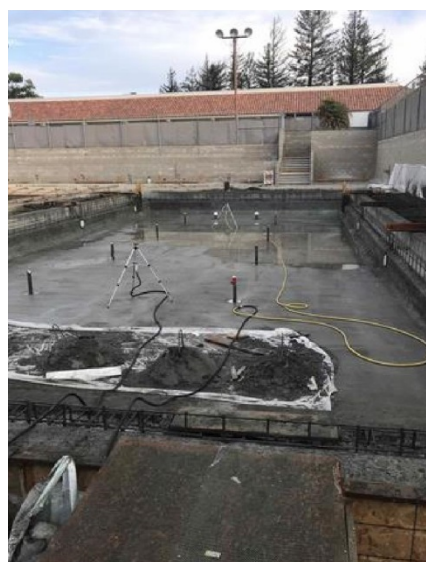
Teaching Pool Shotcrete Cure
