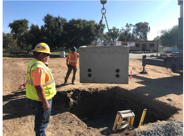
Setting of Electrical/Communication Vault
