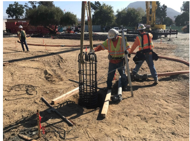
Setting Rebar Cages for Concrete Piers
