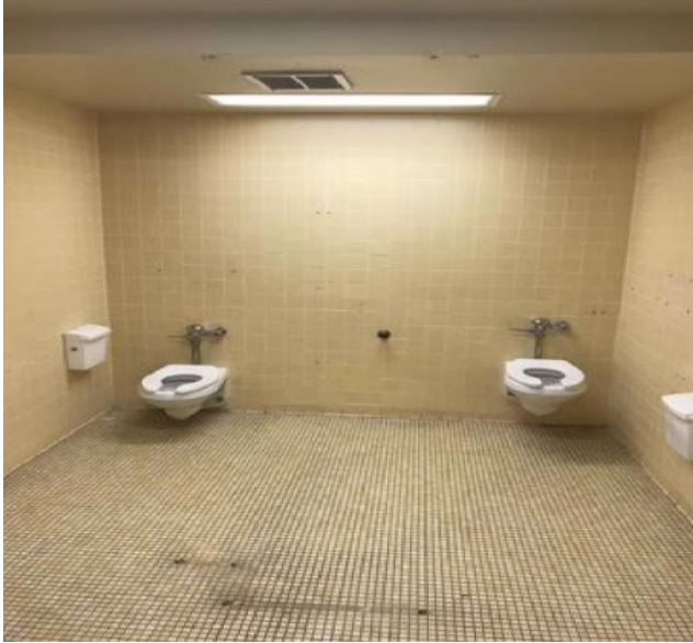
Building 1100 ADA Toilet Demo
