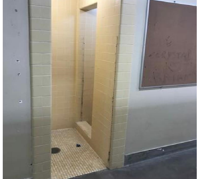
Building 1100 ADA Shower Demo
