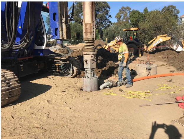
Drilling of Concrete Piers
