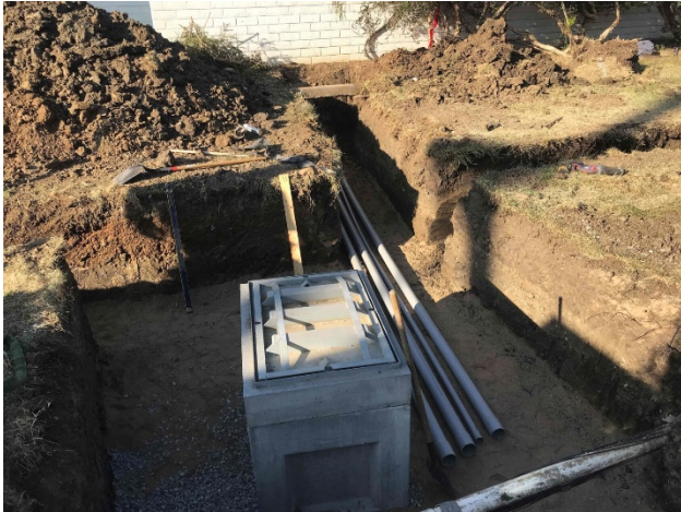
Electrical/Communication Trenching, Conduit and Vault installation progress
