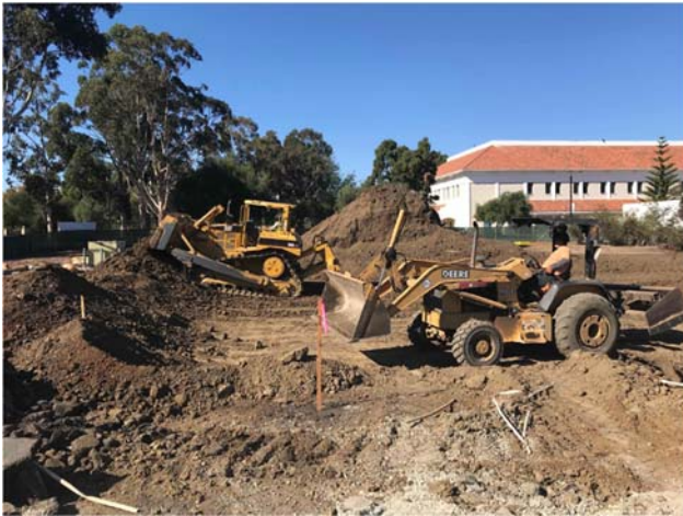
Over-Excavation of Building Pad
