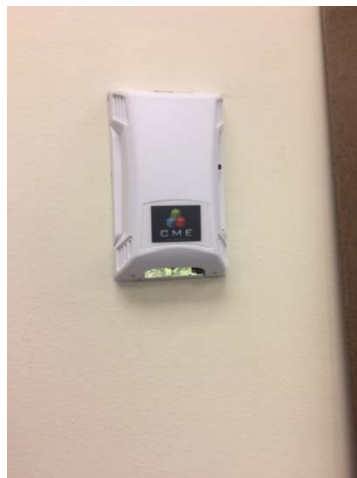
New Thermostats Installed
