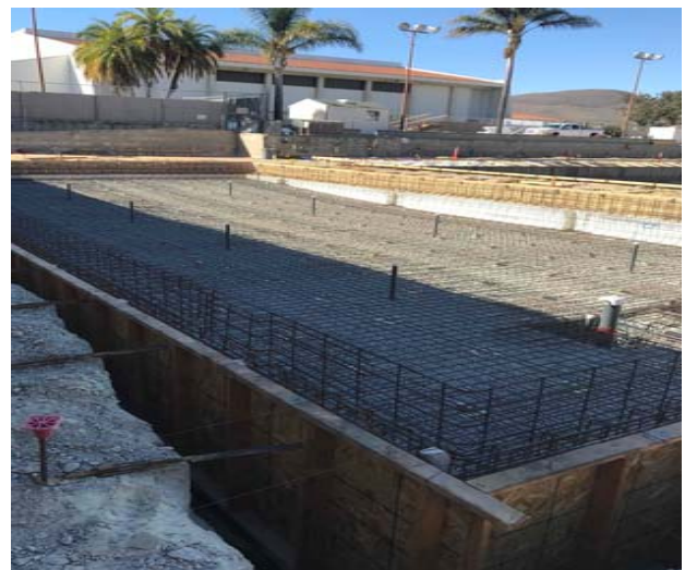
Teaching Pool Reinforcing
