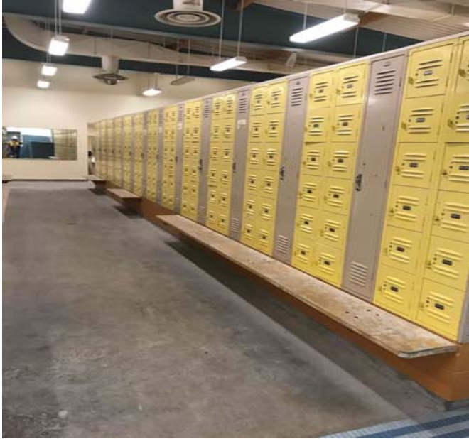
Building 1000 Locker Room Bench Modifications for ADA
