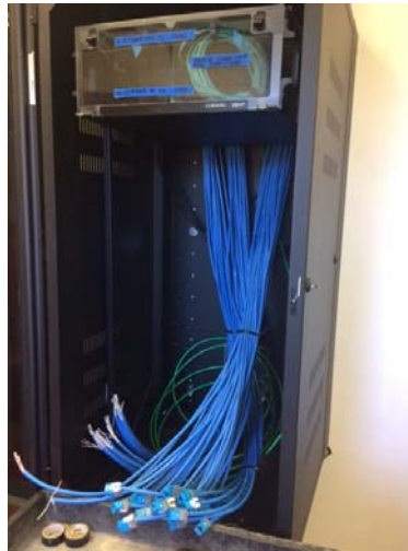
Installation of new IDF Rack and Cabling
