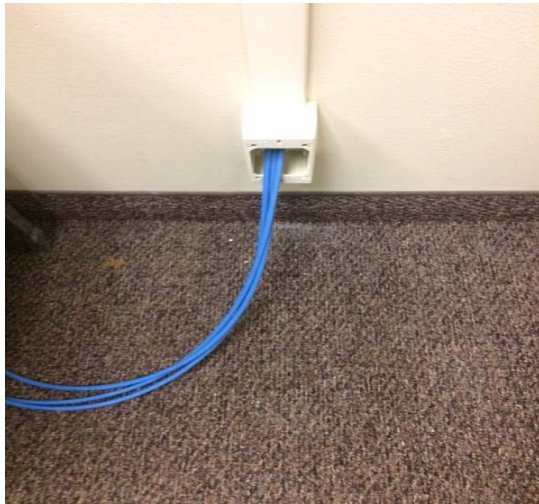
New Data Drops and Cabling
