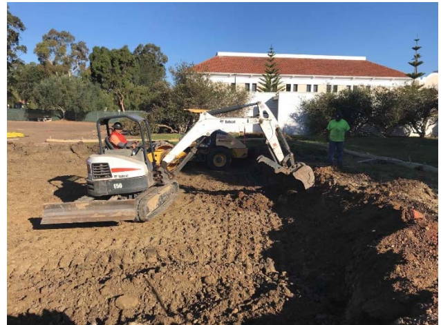
Over-Excavation of Building Pad
