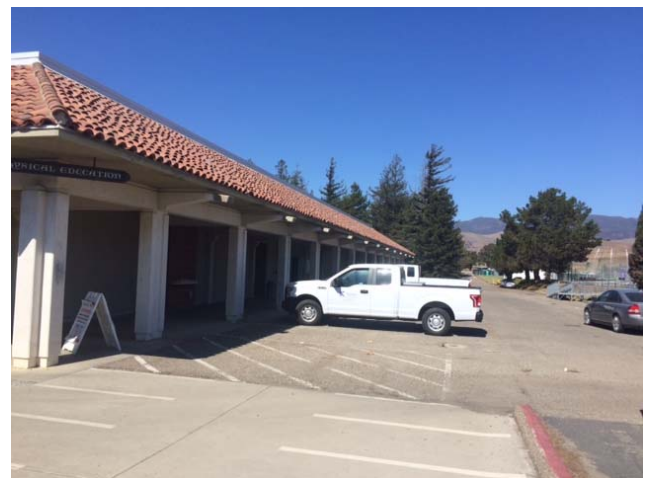
Temporary fencing removed around Buildings 1000 & 1300
