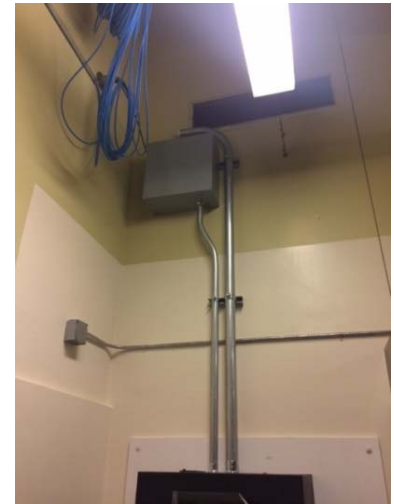
Installation of new raceways
