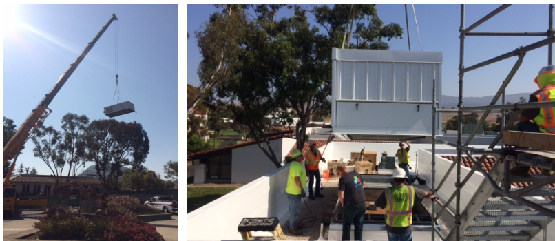
Setting of the mechanical unit on the 1300 Building
