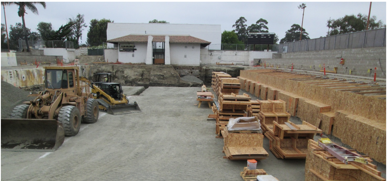
Competition Pool – Formwork & Excavation for Under-slab Piping
