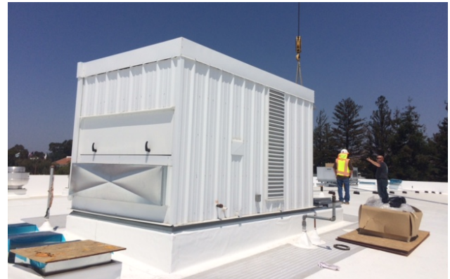
Setting of the mechanical unit on the 1000 Building
