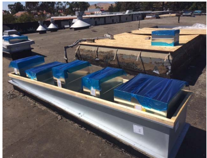
New Duct Penetrations on Building 1000
