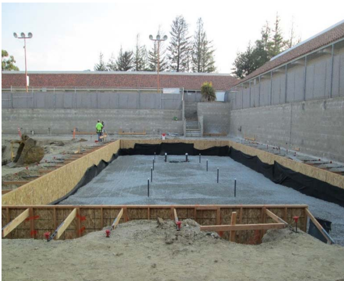
Teaching Pool Below Slab Piping and Subdrain System
