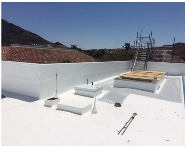
New Roofing on the 1300 Building
