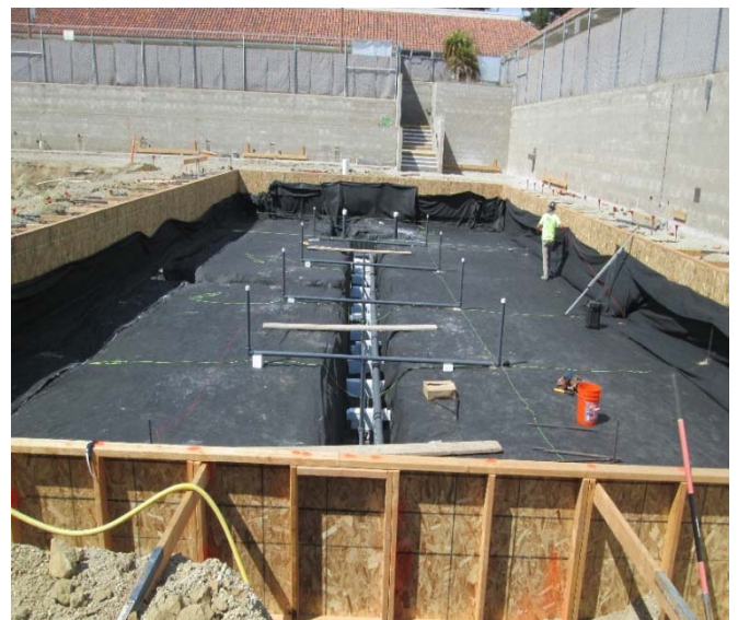
Teaching Pool Below Slab Piping and Subdrain System
