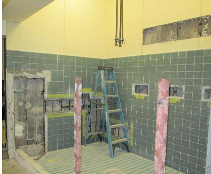
ADA Restroom Upgrade Selective Demo
