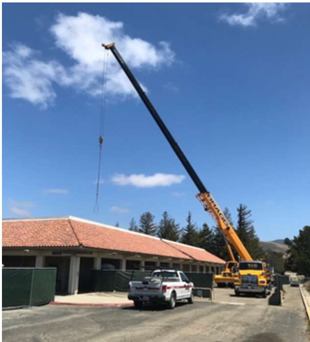
Removal of Existing HVAC Units
