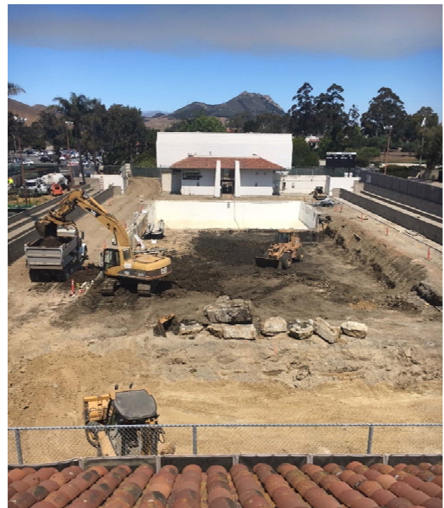
Excavation for Competition Pool
