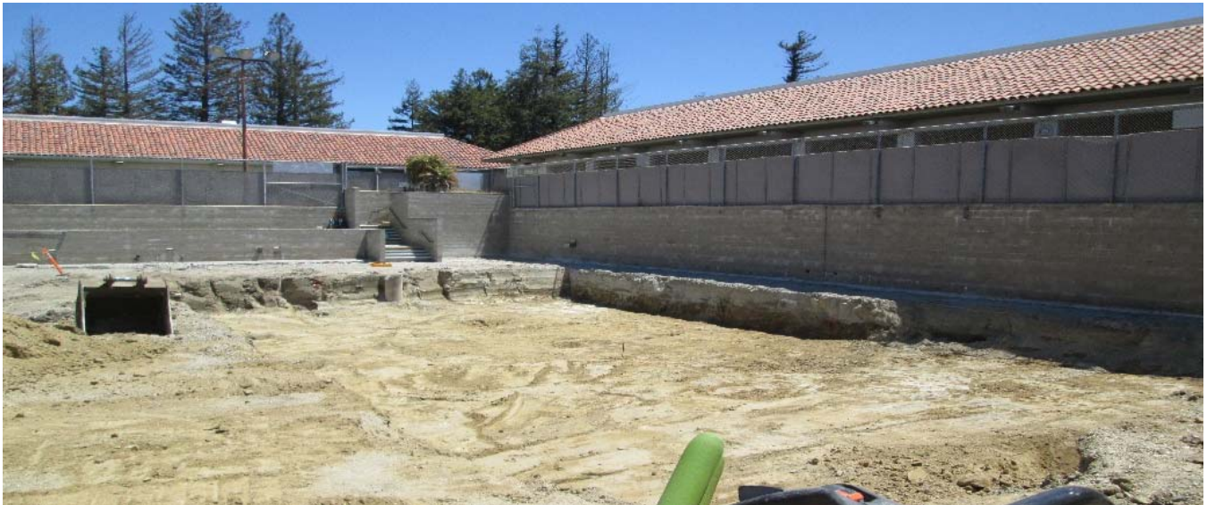
Pools Drained and Soft Demo Started
