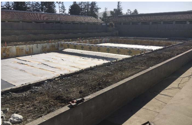
Pools Drained and Soft Demo Started
