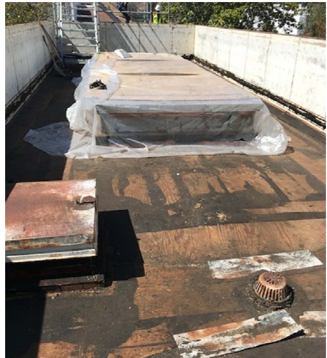
Demolition of the Existing Roofing
