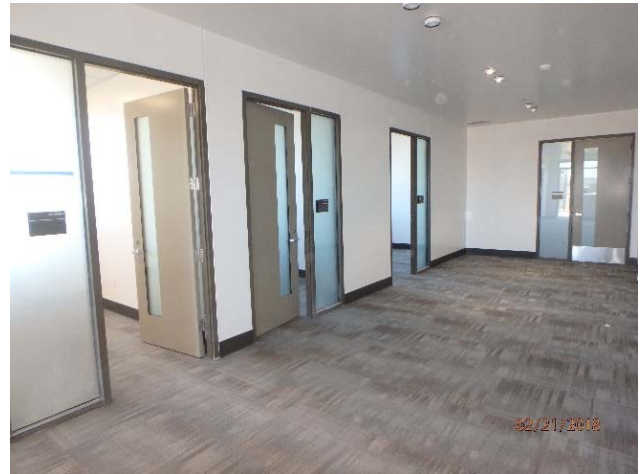
Carpet Installed on the Second Floor
