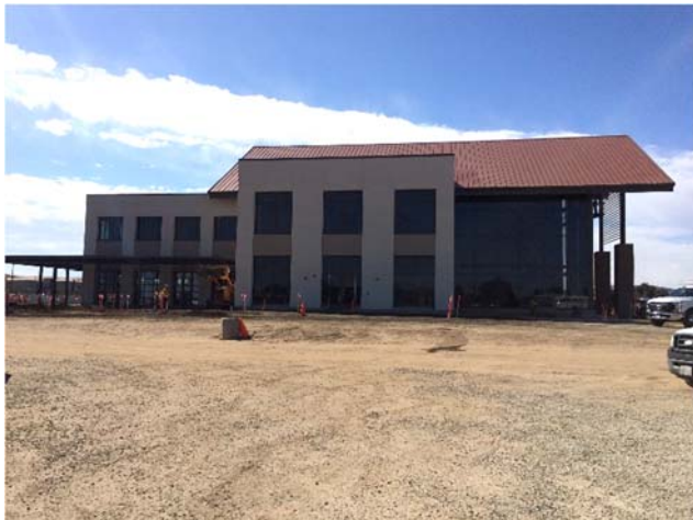
Sitework Grading Progress
