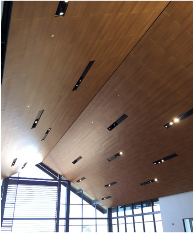
Torsion Spring High Ceiling Installation
