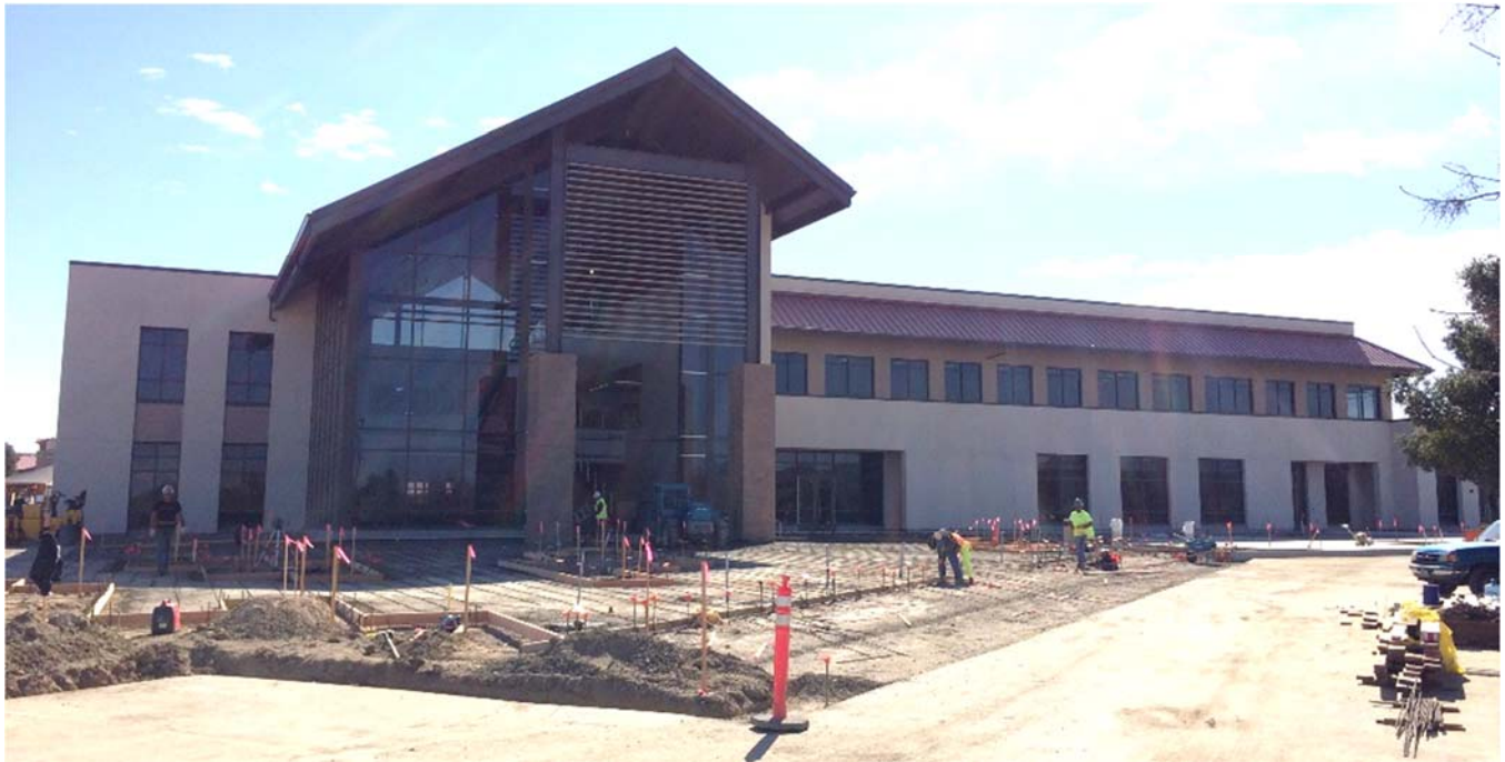
Forming for Site Concrete
