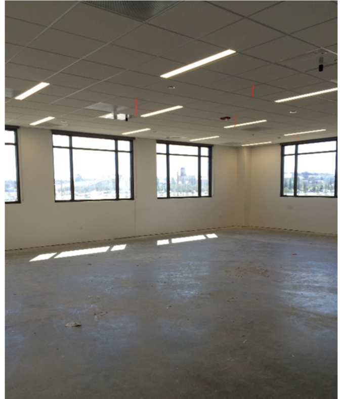
Classroom ready for Flooring
