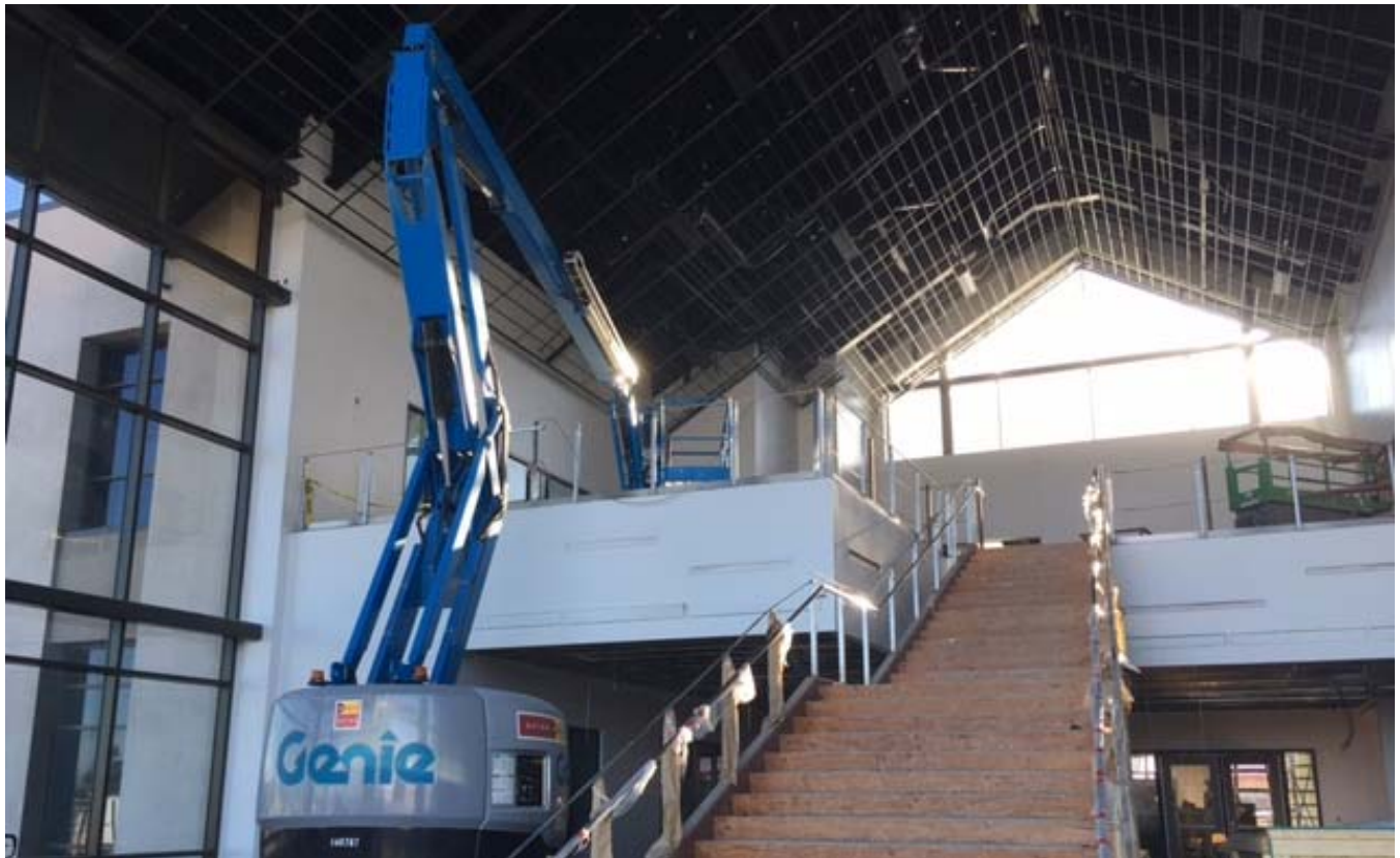
Progress on Torsion Spring Acoustical Ceiling Grid Installation
