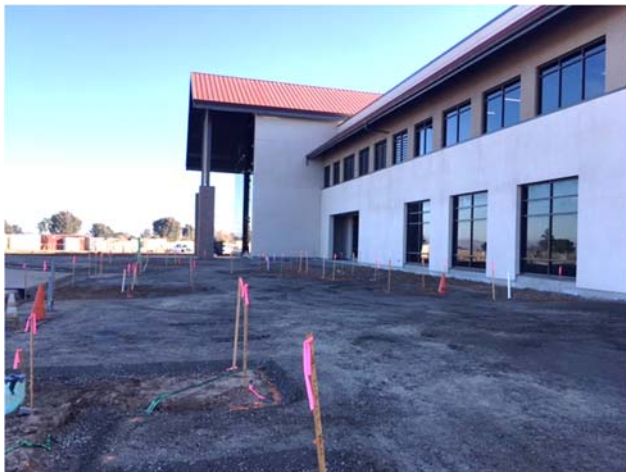
Sitework Grading Progress in Preparation for Concrete
