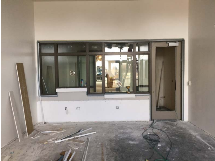
Safety Glass Windows at Public Safety Service Counter
