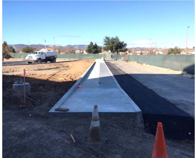
Completed Concrete ADA Walkway at Parking Lot 10
