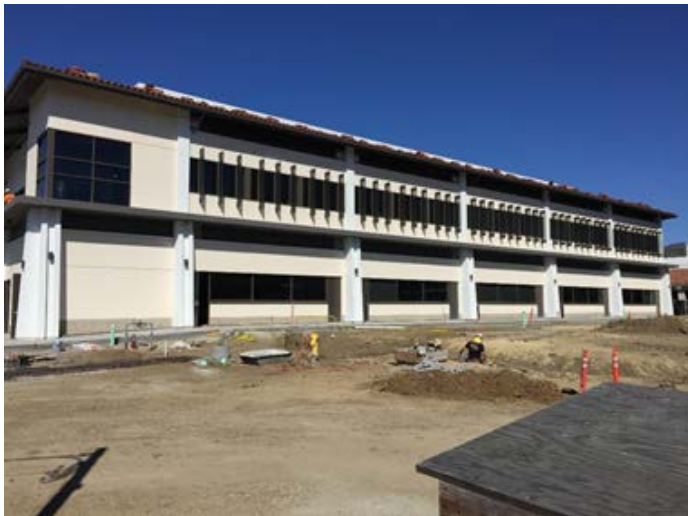
Building Exterior with Site Work
