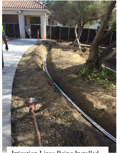
Irrigation Lines Being Installed
