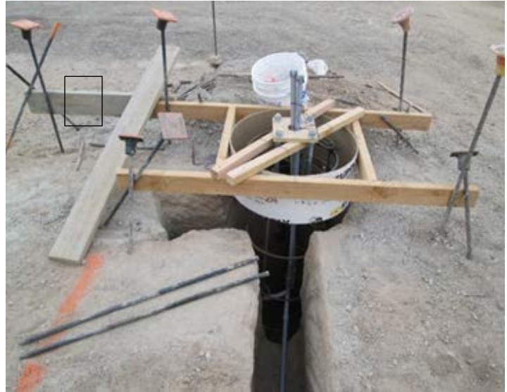
Foundation Preparation for Site Lighting
