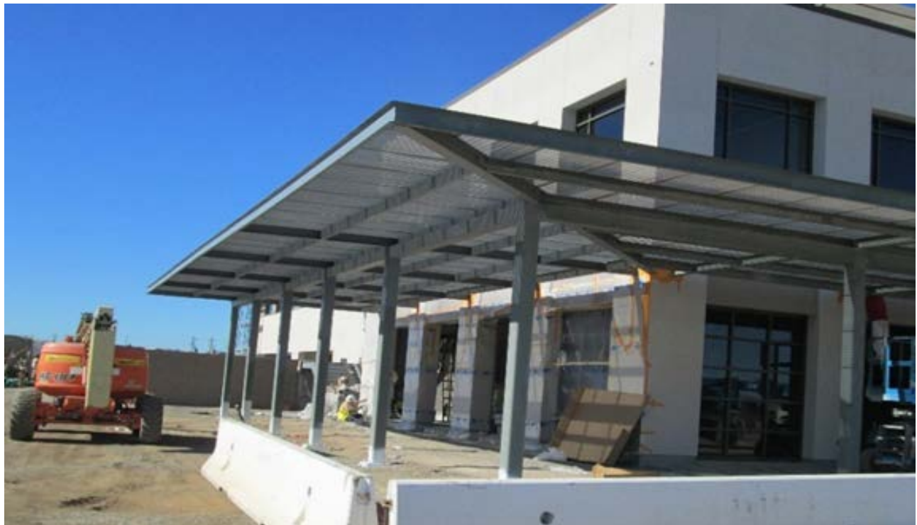
Metal Panels Installed on Trellis Roof
