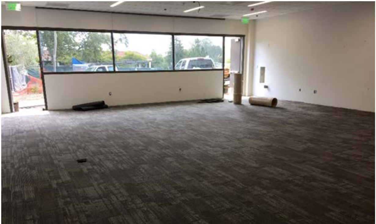
First Floor Classroom Carpet Installation
