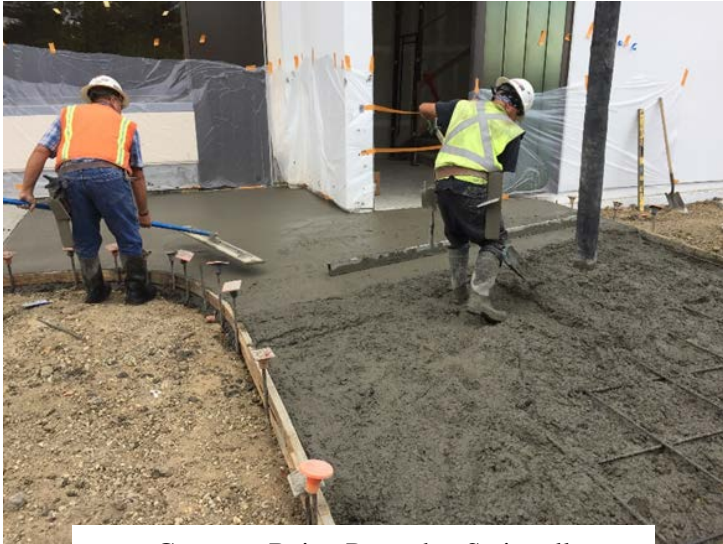
Concrete Being Poured at Stairwell
