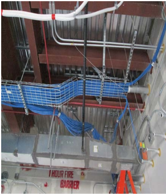
Above Ceiling Installations
