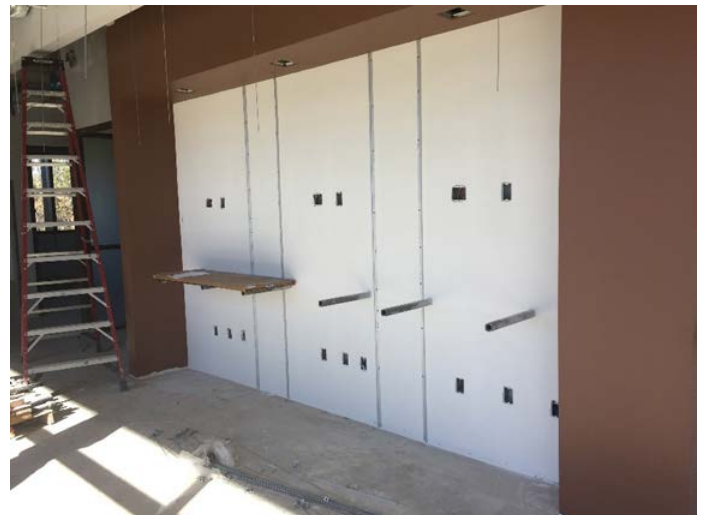
Computer Station on Second Floor
