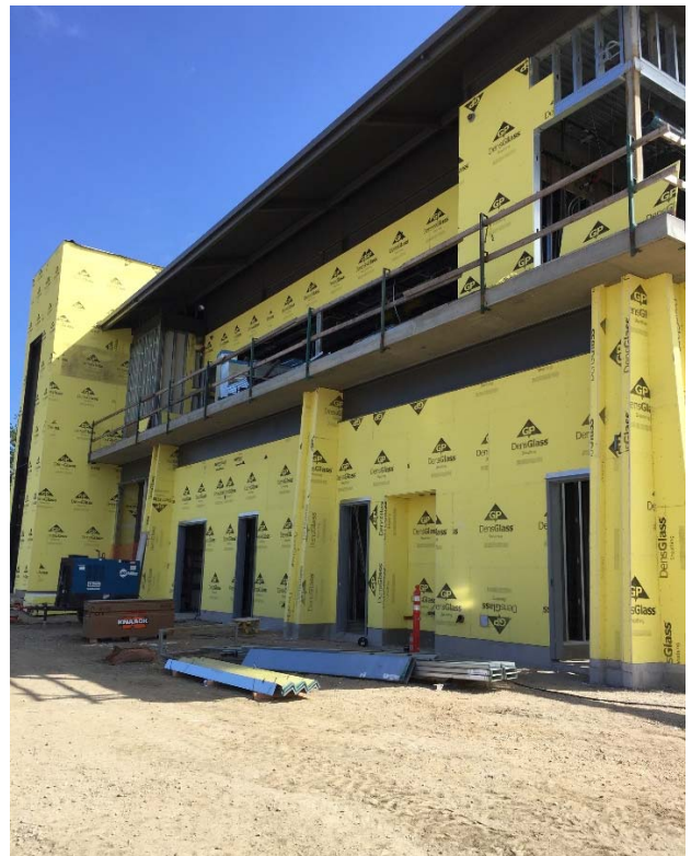
Exterior Columns with Sheathing in Place
