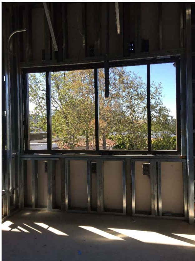
Second Floor Window Installation
