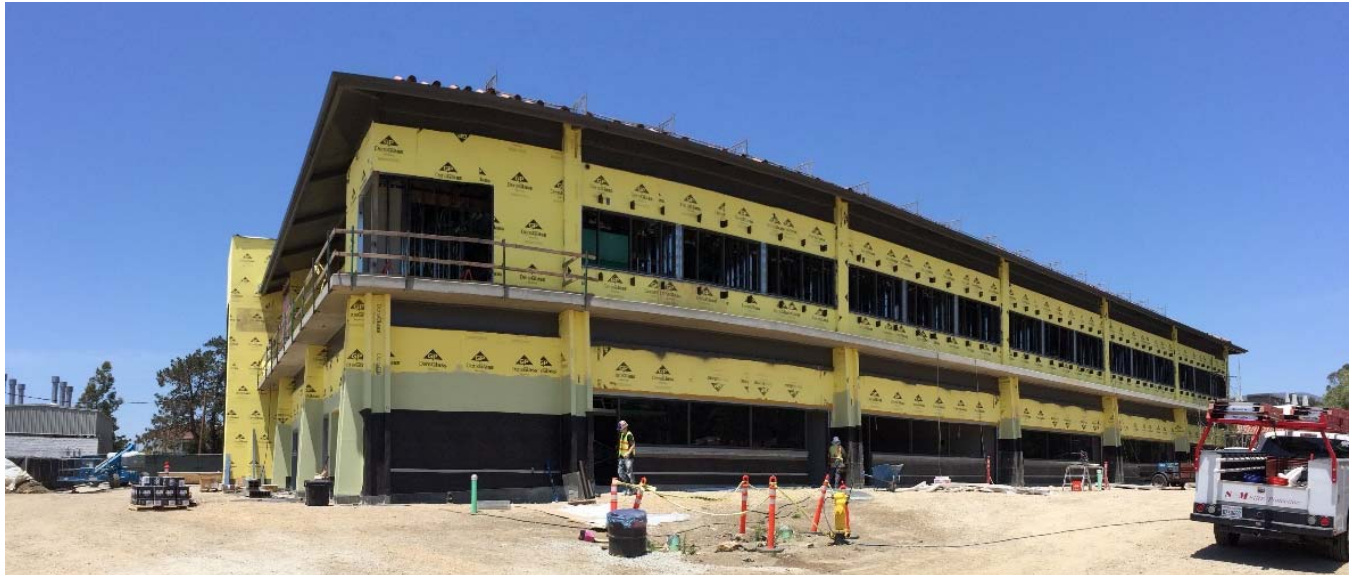
Exterior Progress from the Northwest Corner
