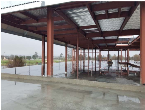
Second Floor Concrete Deck
