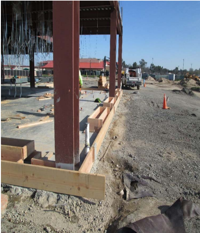
Formwork for Perimeter Curbs
