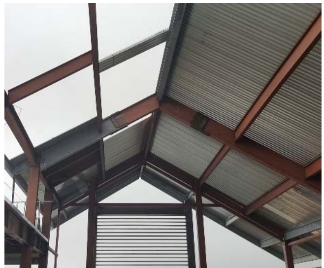
Decking at High Roof
