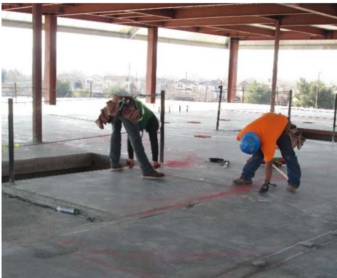
Layout for Interior Wall Framing
