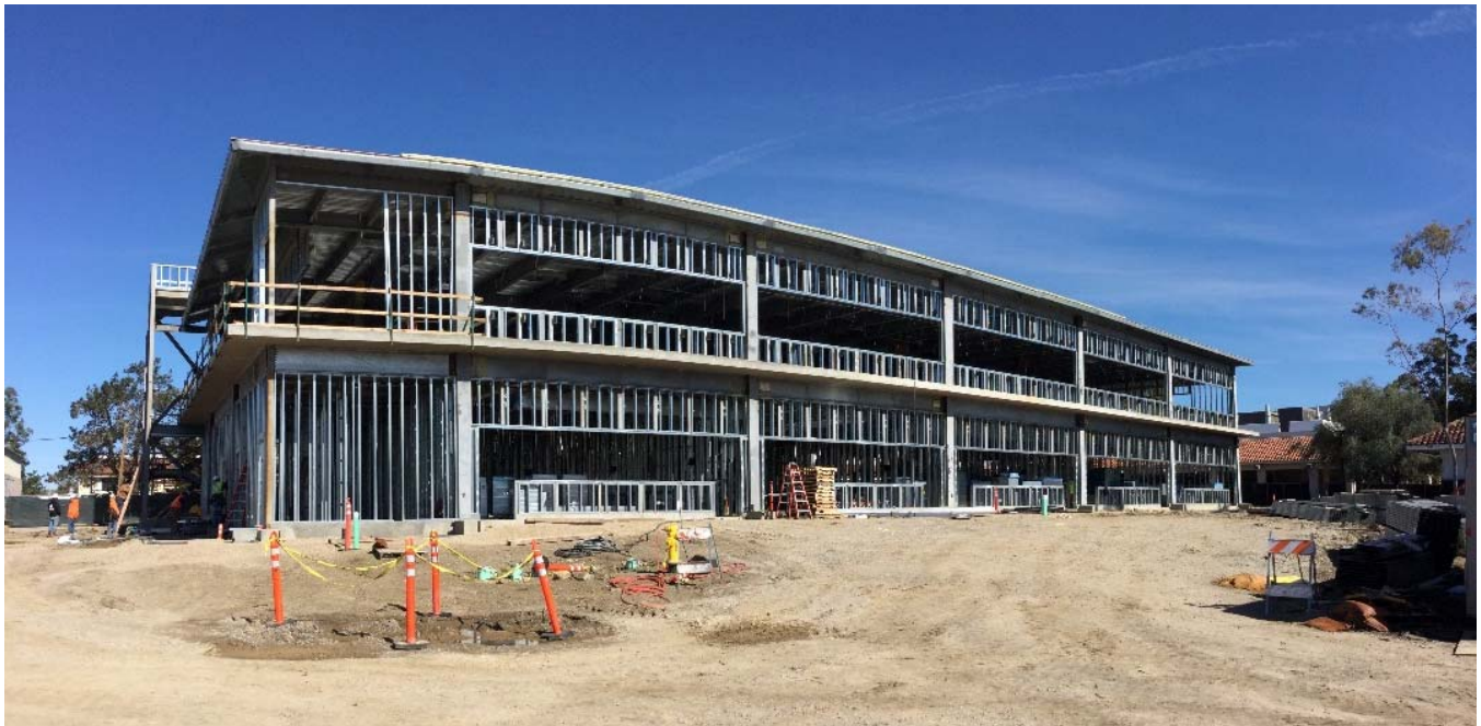
Exterior Framing Progress on the Southside of the Building
