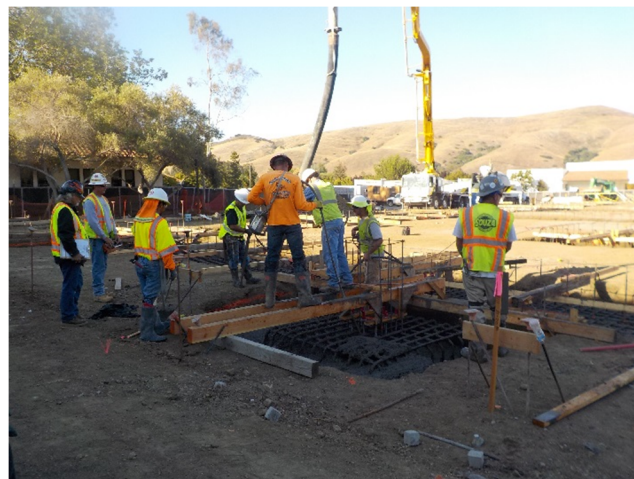
Concrete Placement of Structural Footings
