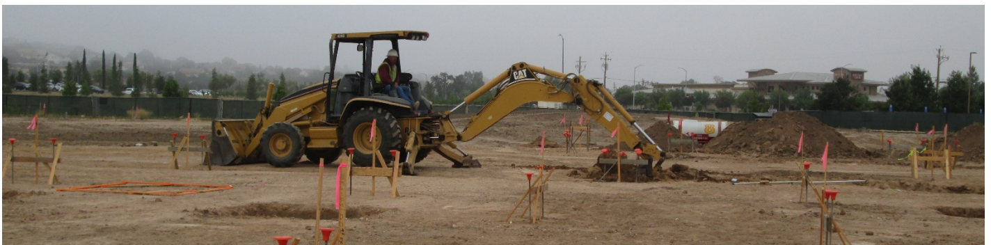
Excavation of Footings & Grade Beams
