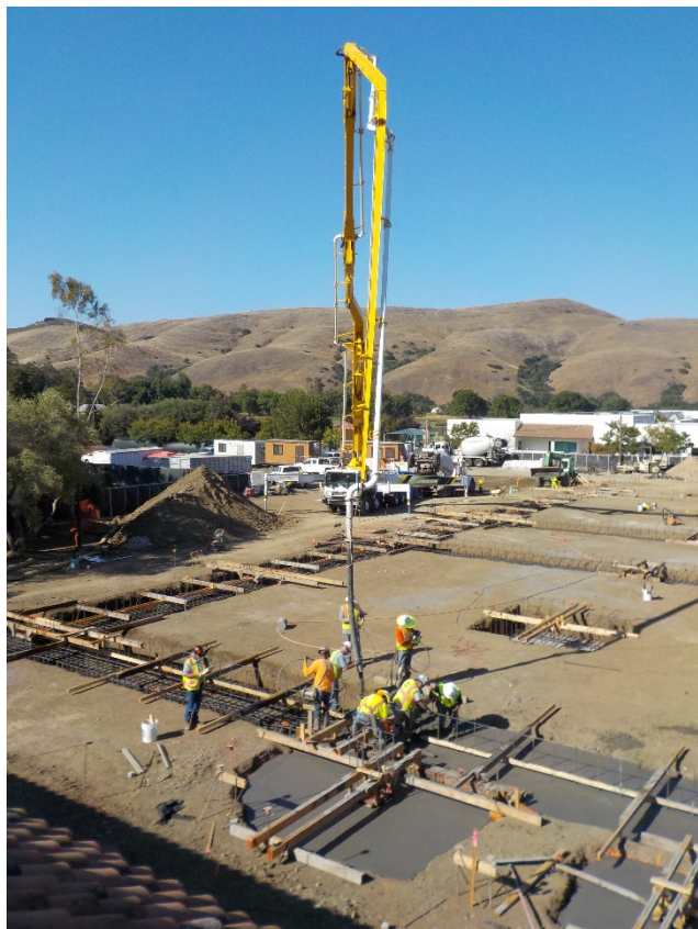
Concrete Placement of Structural Footings
