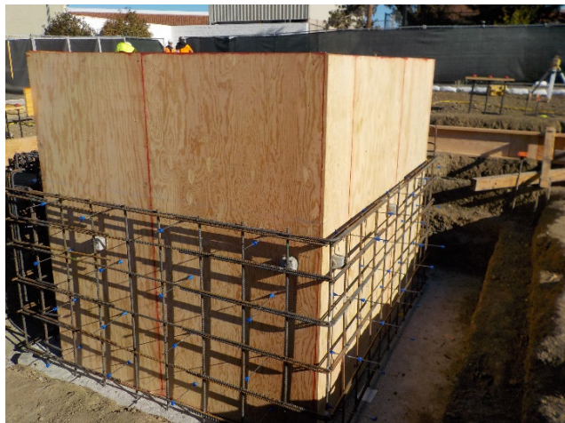
Steel Reinforcing at Elevator Pit Walls
