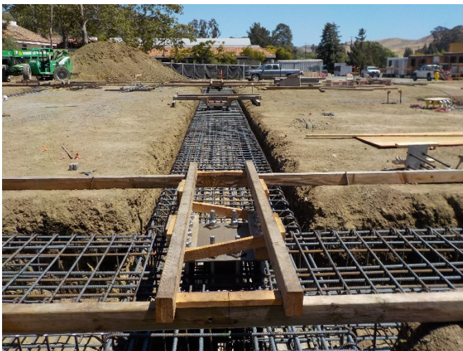
Steel Reinforcing and Anchor Bolts at Interior Building Grade Beam
