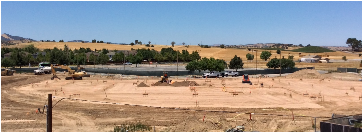
Start of Footing & Grade Beam Excavation
