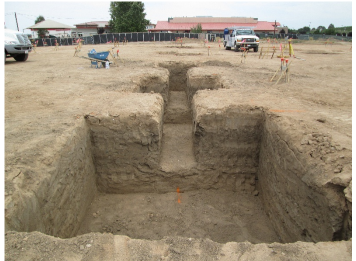
Excavation of Footings & Grade Beams
