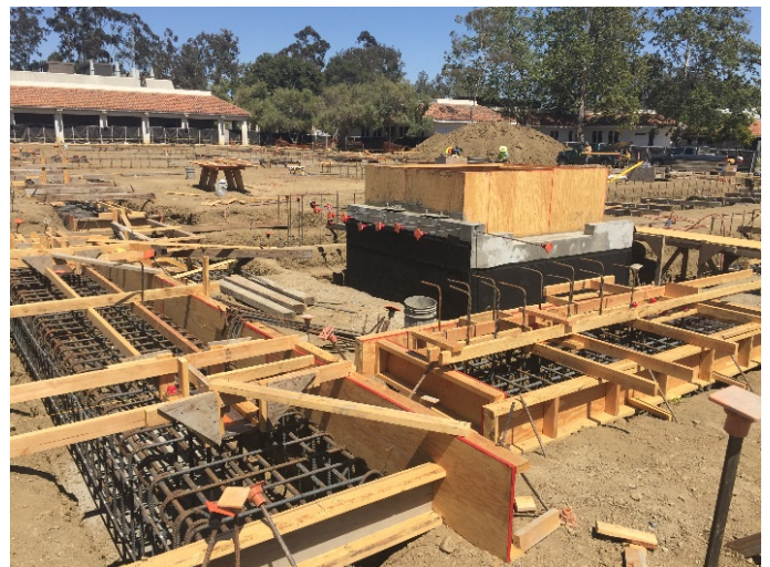
Formwork at New Elevator Pit
