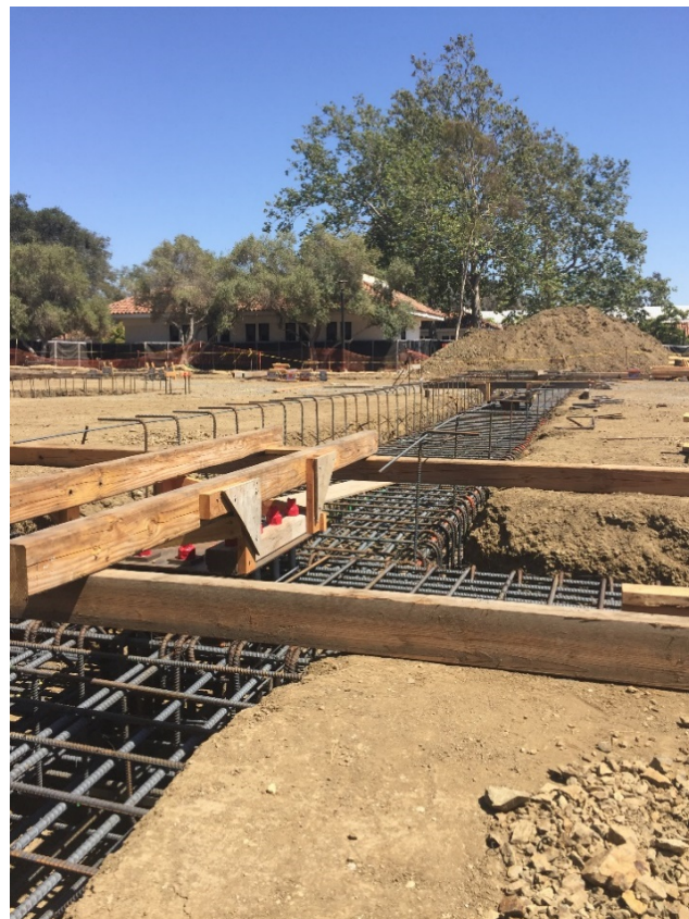
Steel Reinforcement at Footings
