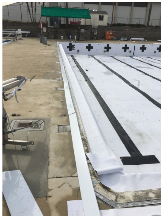
Pool Liner Installation
