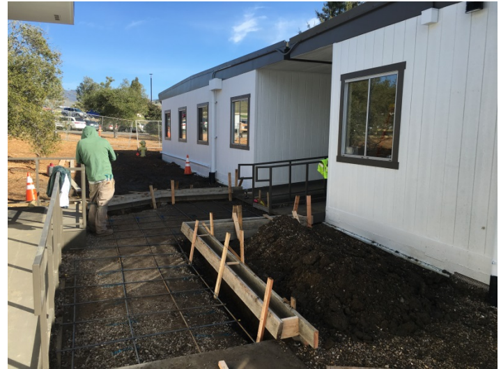
Preparation for Concrete Walkways
