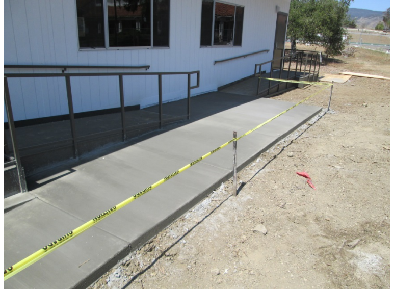
Public Safety/Staff Offices Portable Access
