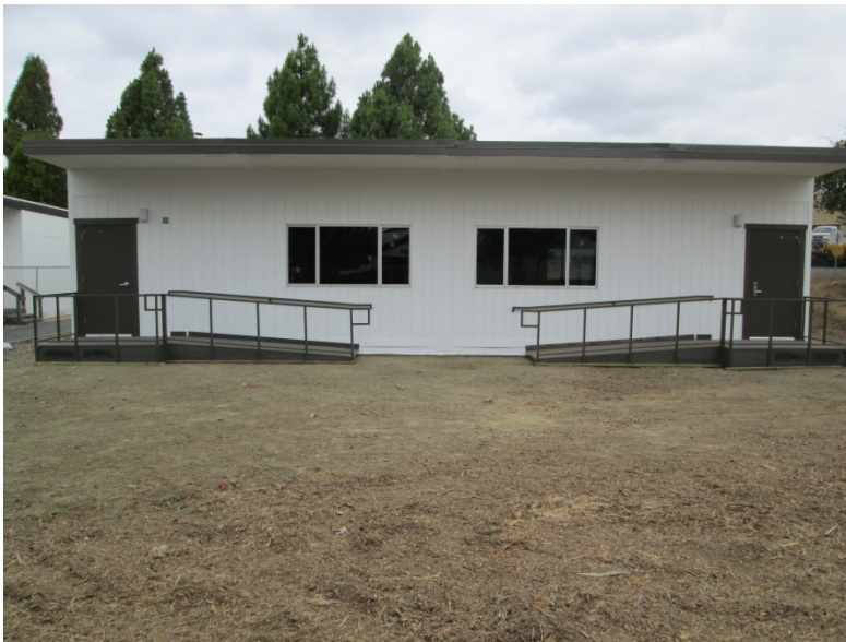
Public Safety Portable Building
