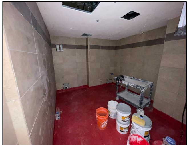
Plaster Installed In Preparation for Tile
