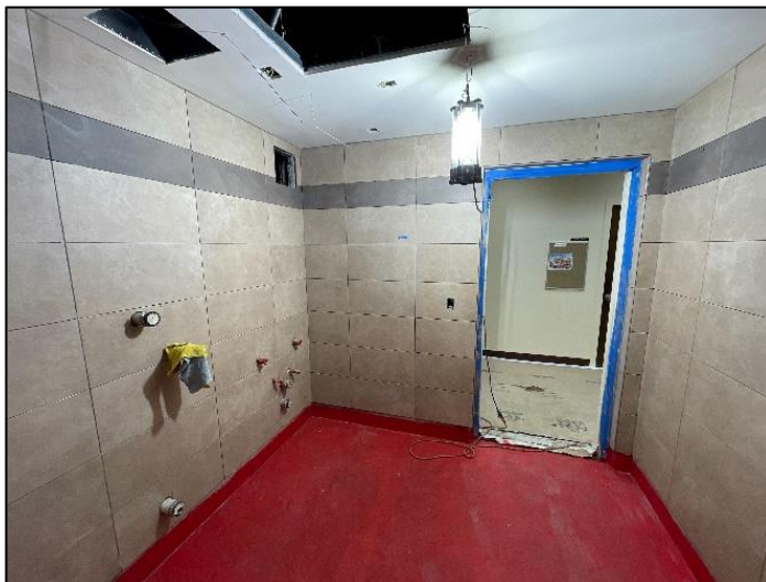
Vapor Barrier In Preparation for Lath
