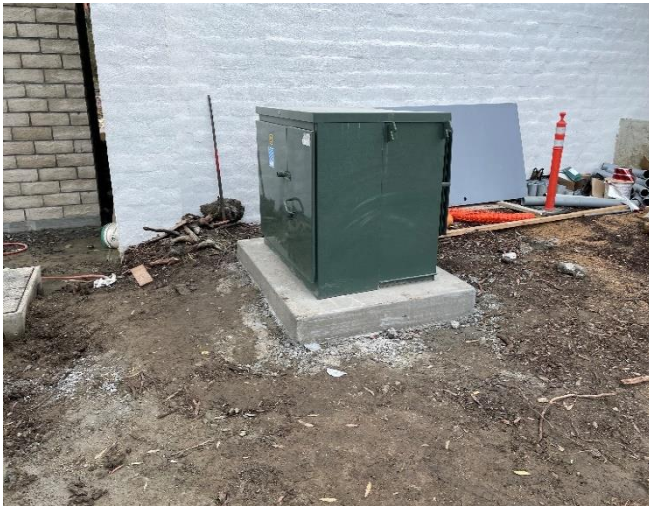
Temp Transformer & Pad
