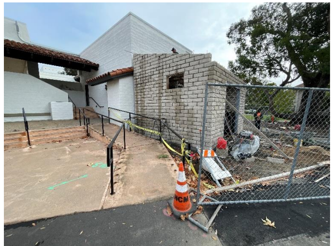
Completion of Block Structure
