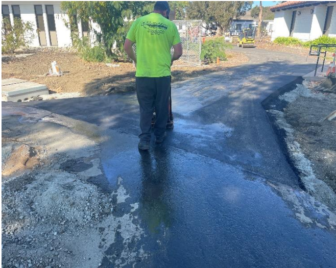
Pavement patch at walkway
