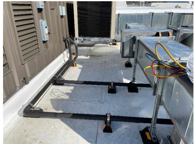
New Refrigerant Piping
