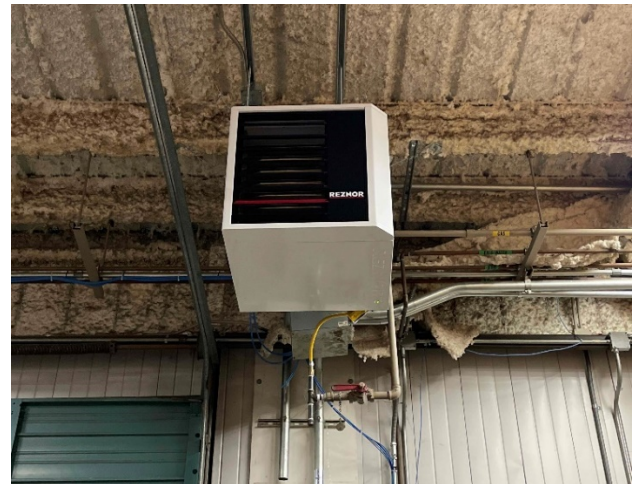
New Heater in Groundskeeping Area
