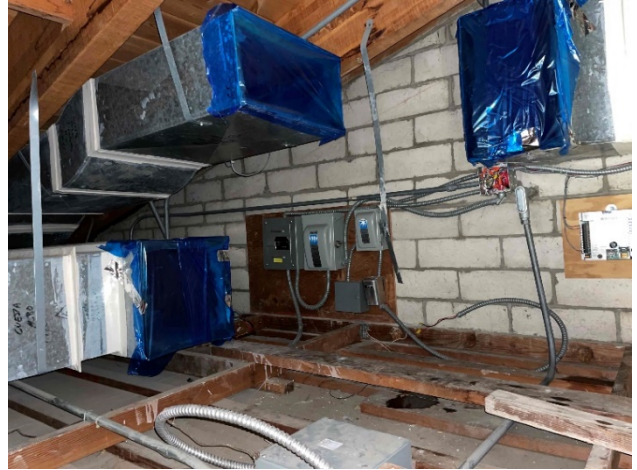
Ductwork Inside Building
