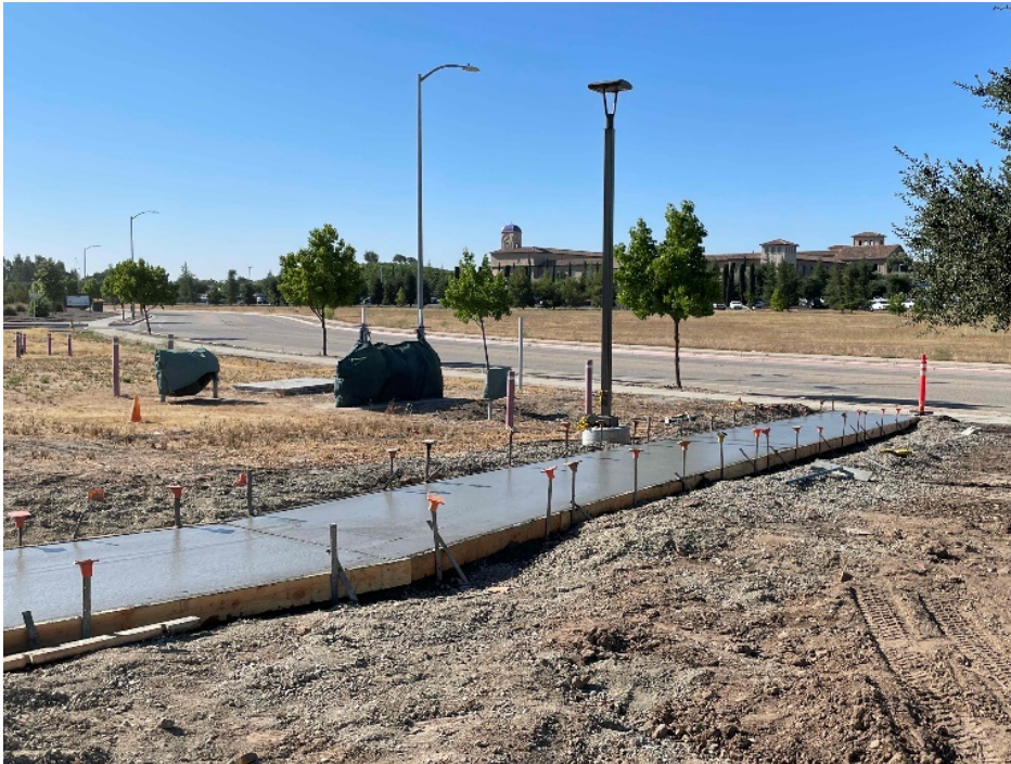
Concrete Placement at New Walkways
