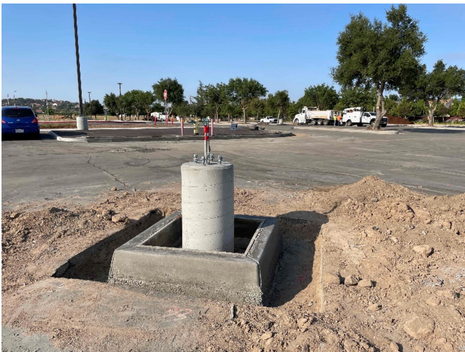
New Site Lighting Pole Bases Complete
