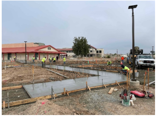
Concrete Placement in Progress
