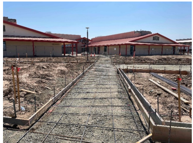
Concrete Formwork Installation Progress
