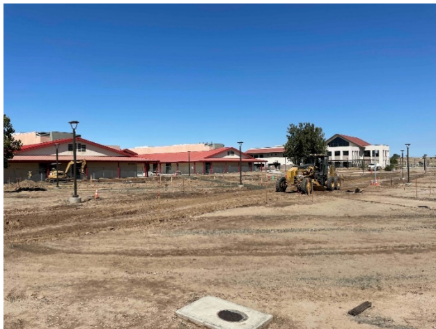
Site Grading, Base Placement and Compaction Progress
