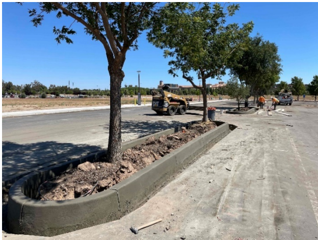
New Concrete Curb Installation Progress
