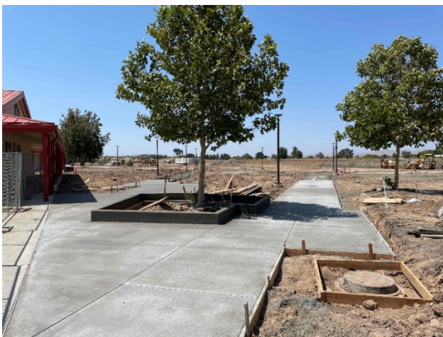
Completed Concrete Walkways
