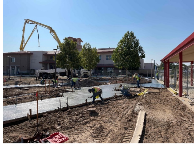
Concrete Placement in Progress
