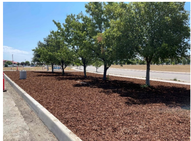
New Bark Installation Progress at Perimeter Planter Areas
