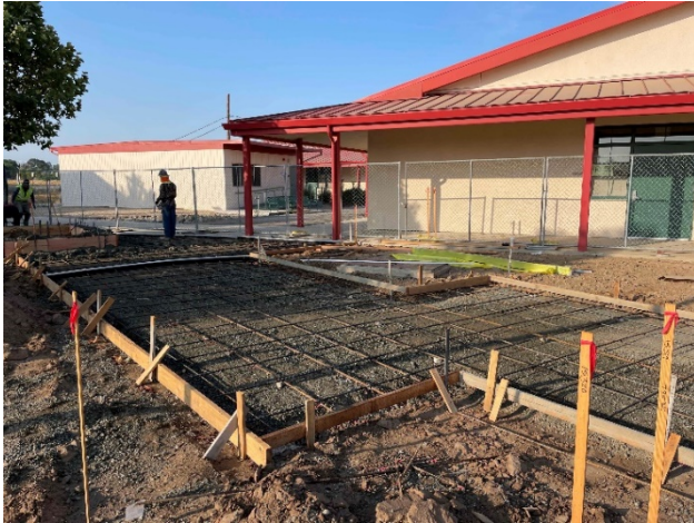
Concrete Formwork Installation Progress
